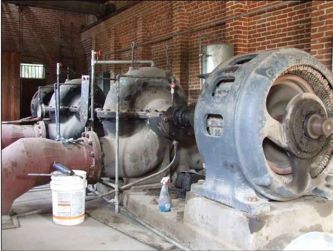
Photograph 15 of 25 Interior, view looking NW
