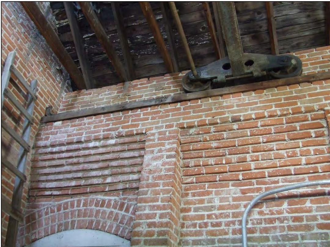
Photograph 18 of 25 Pulley rail, corbelled wall and segmental arch, north wall
