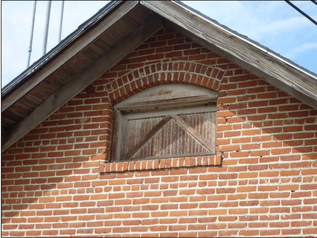
Photograph 7 of 25 Detail view, segmental arch and window, façade
