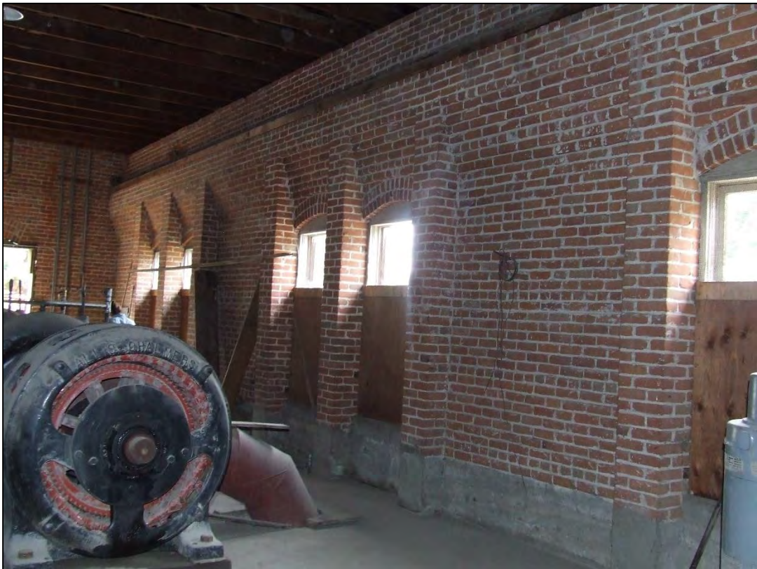
Photograph 20 of 25 South wall, view looking SE
