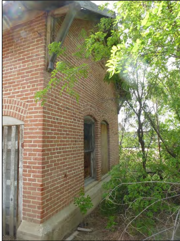
Photograph 11 of 25 West elevation, view looking S
