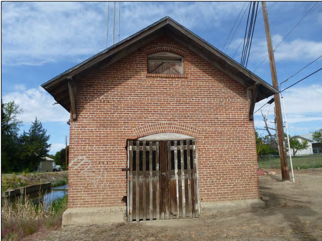
Photograph 2 of 25 Façade (east elevation), view looking W
