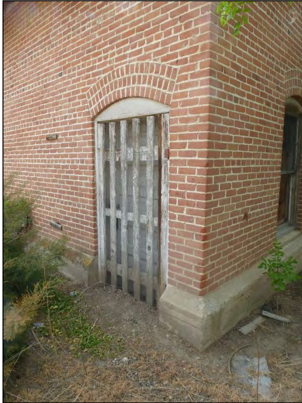
Photograph 9 of 25 Door, north elevation
