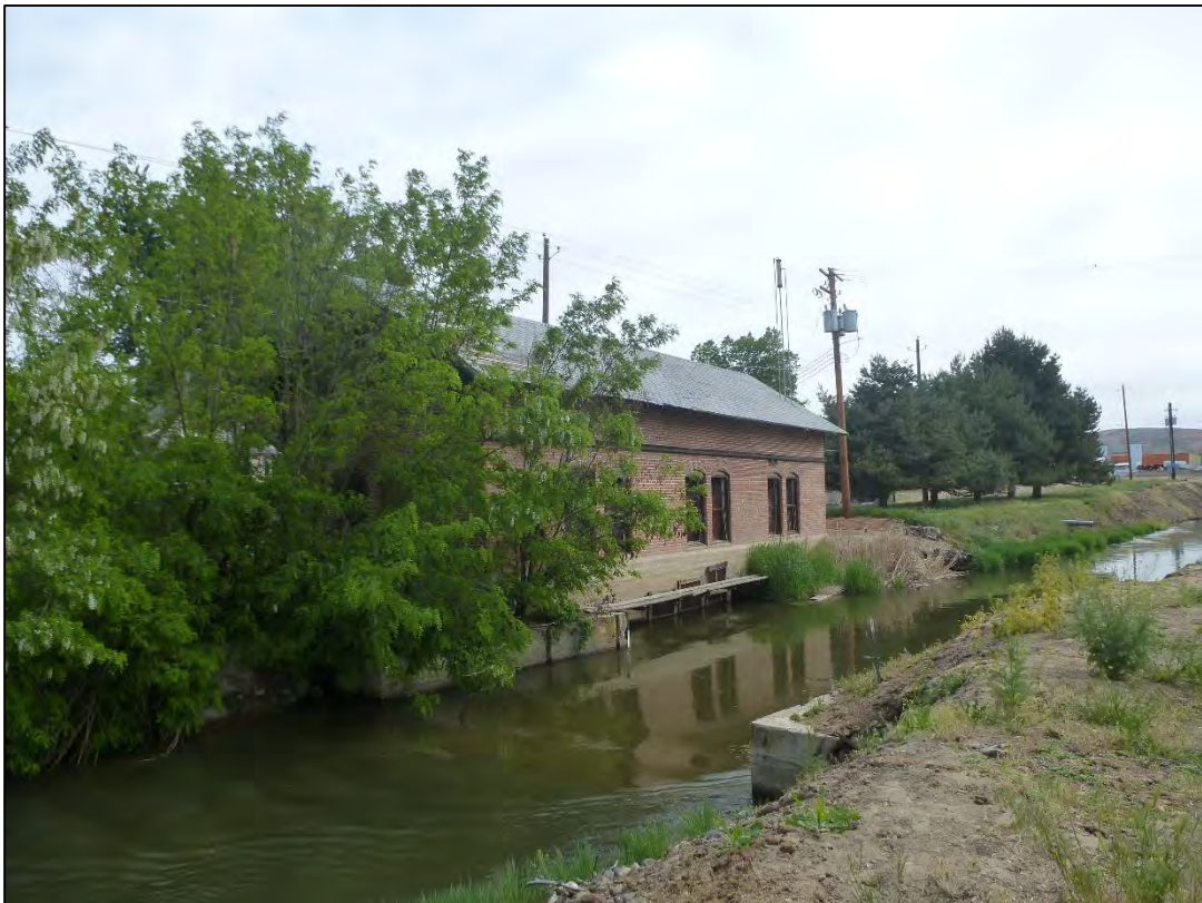
Photograph 6 of 25 South elevation, view looking NE
