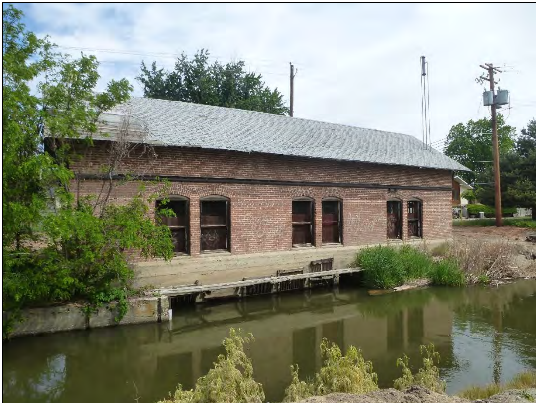
Photograph 12 of 25 South elevation, view looking NE
