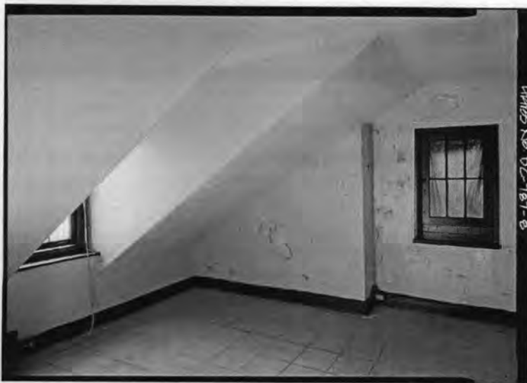
604 H Street NW, Washington, DC, Fourth Floor, Front Room 1988. Boucher, Jack. Historic American Building Survey, Library of Congress Prints and Photographs Division
