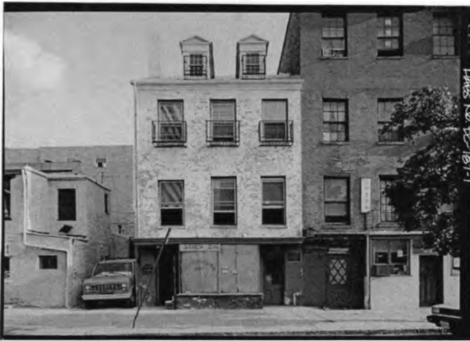
604 H Street NW, Washington, DC, North Front Façade, 1988. Boucher, Jack. Historic American Building Survey, Library of Congress Prints and Photographs Division.
