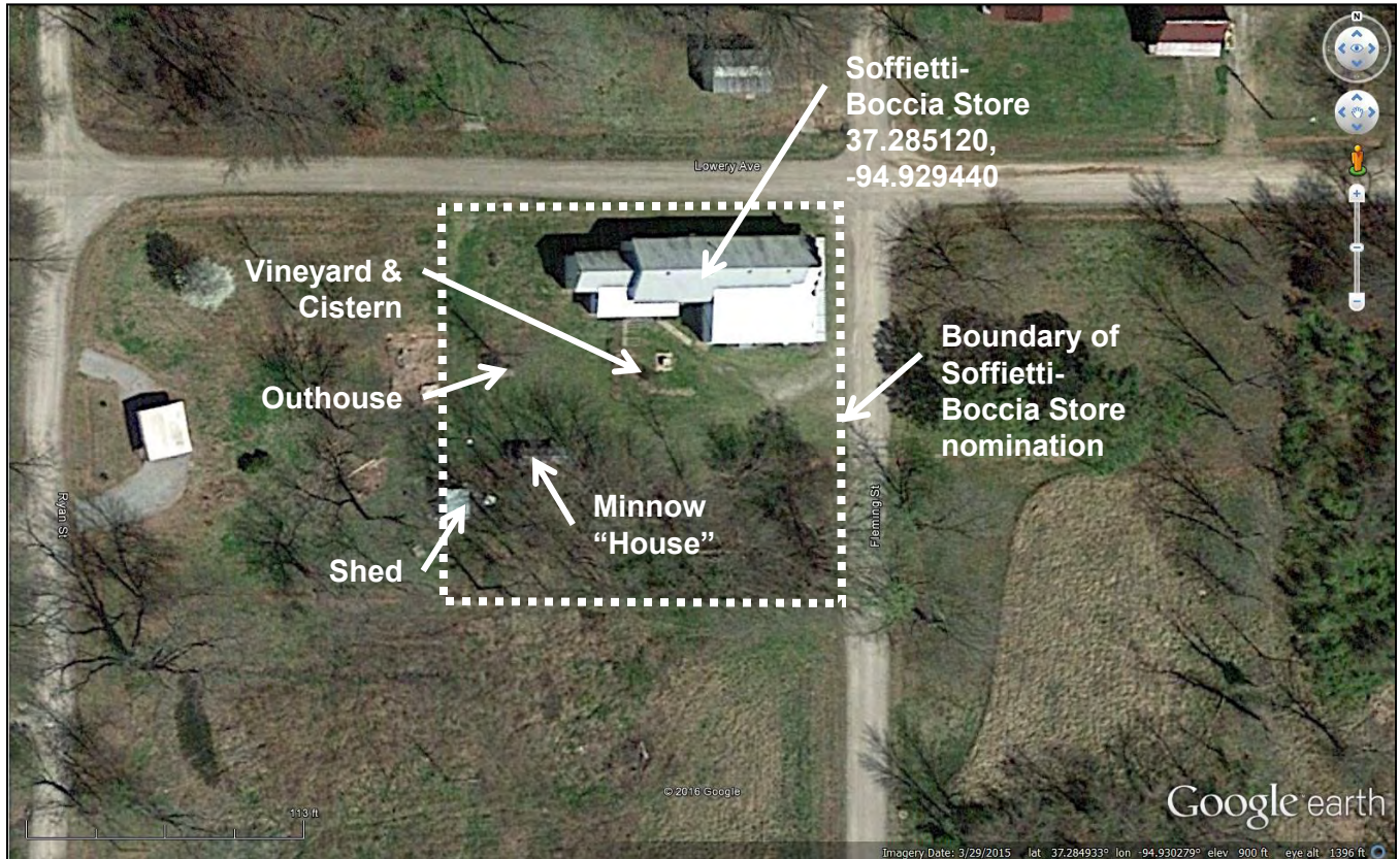
Figure 2 (Boundary Map). 2015 Google aerial image of Soffietti-Boccia Store boundary.
