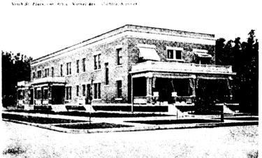
one-over-one double hung wood sash and appear in single and paired configurations. The perimeter of the upper façade is decorated with a pressed tin cornice band with a fleur-de-lis pattern. Carthage Stone stringcourses separate the concrete foundation, and the water-table, and the body of the structure. The historic post card (above) shows a balustrade at the top of the main porch roof and side porches. These railings are no longer extant.
