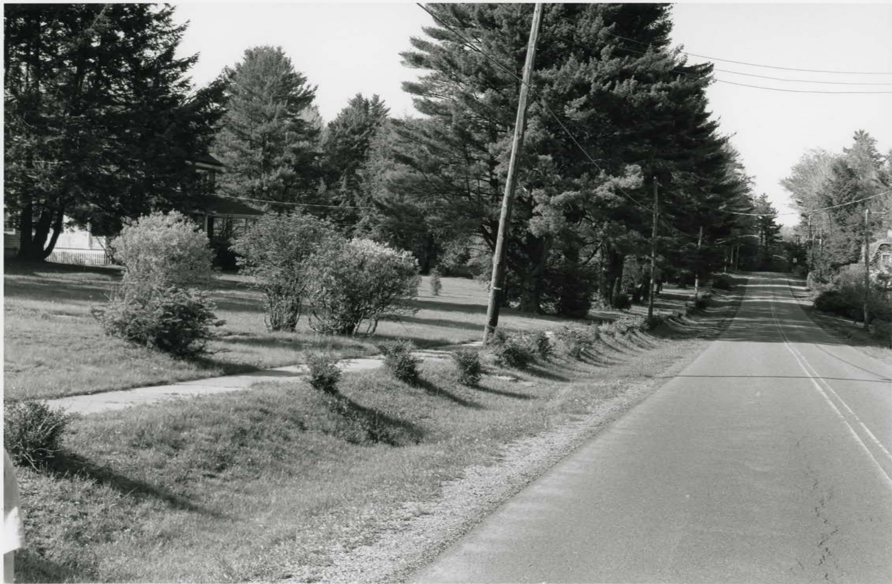
Pennsylvania Avenue, Eagles Mere Historic District Sullivan County, PA
