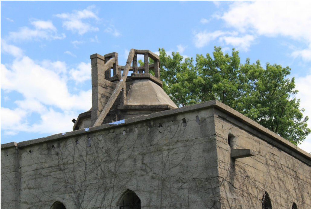
7 of 22: Cornice and Upper Wall Detail, Northwest Corner. Camera looking southeast.
