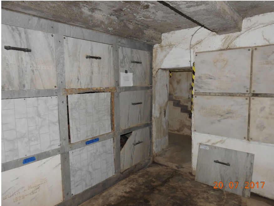
11 of 22: Front Crypt Room, First Floor. Camera looking northwest.
