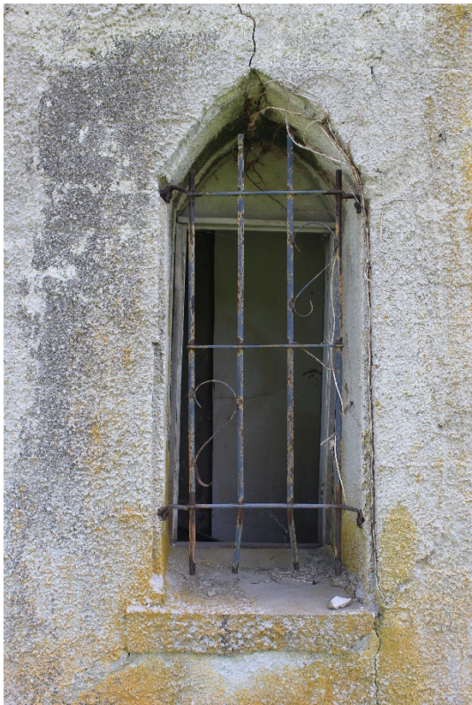
5 of 22: Window Detail, North Side. Camera looking south.
