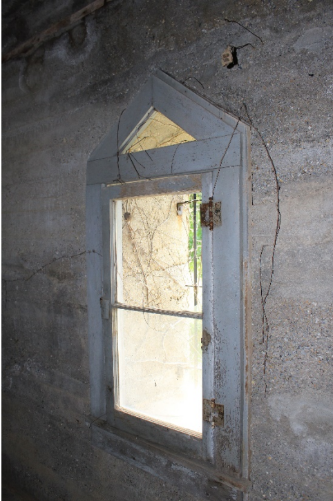
21 of 22: Interior Window Detail, Museum Room, Second Floor. Camera looking southwest.
