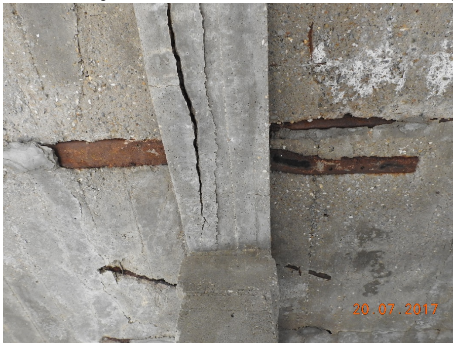
20 of 22: Ceiling Detail, Museum Room, Second Floor. Camera looking up.
