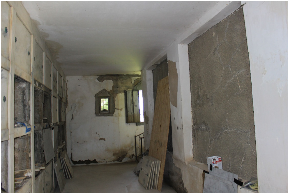
13 of 22: Back Crypt Room, First Floor. Camera looking north.
