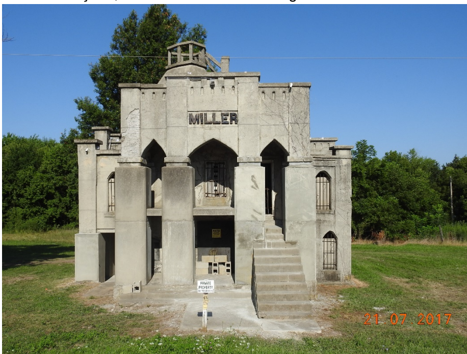
2 of 22: Façade, East side. Camera looking west.
