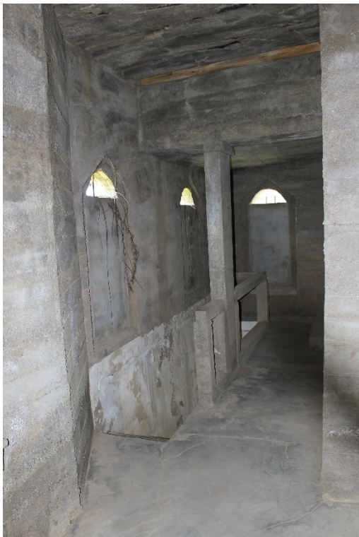
14 of 22: North Hall, Second Floor. Camera looking east.
