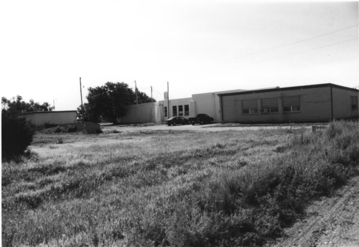
SHALLOW WATER SCHOOL, SCOTT COUNTY, KANSAS #6
