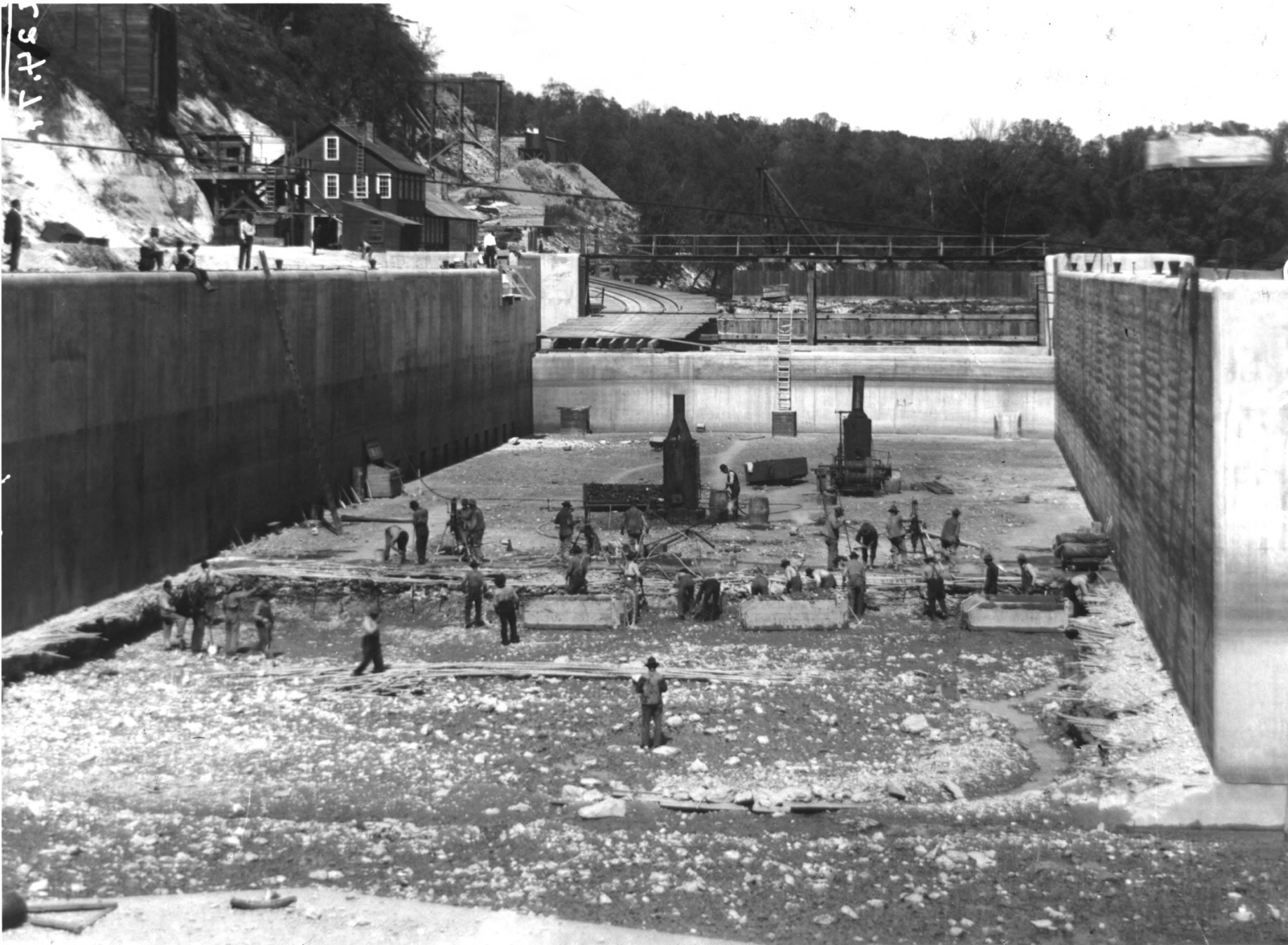
Lock and Dam No. 2 Hennepin and Ramsey Counties, Minnesota MHS 6994A
