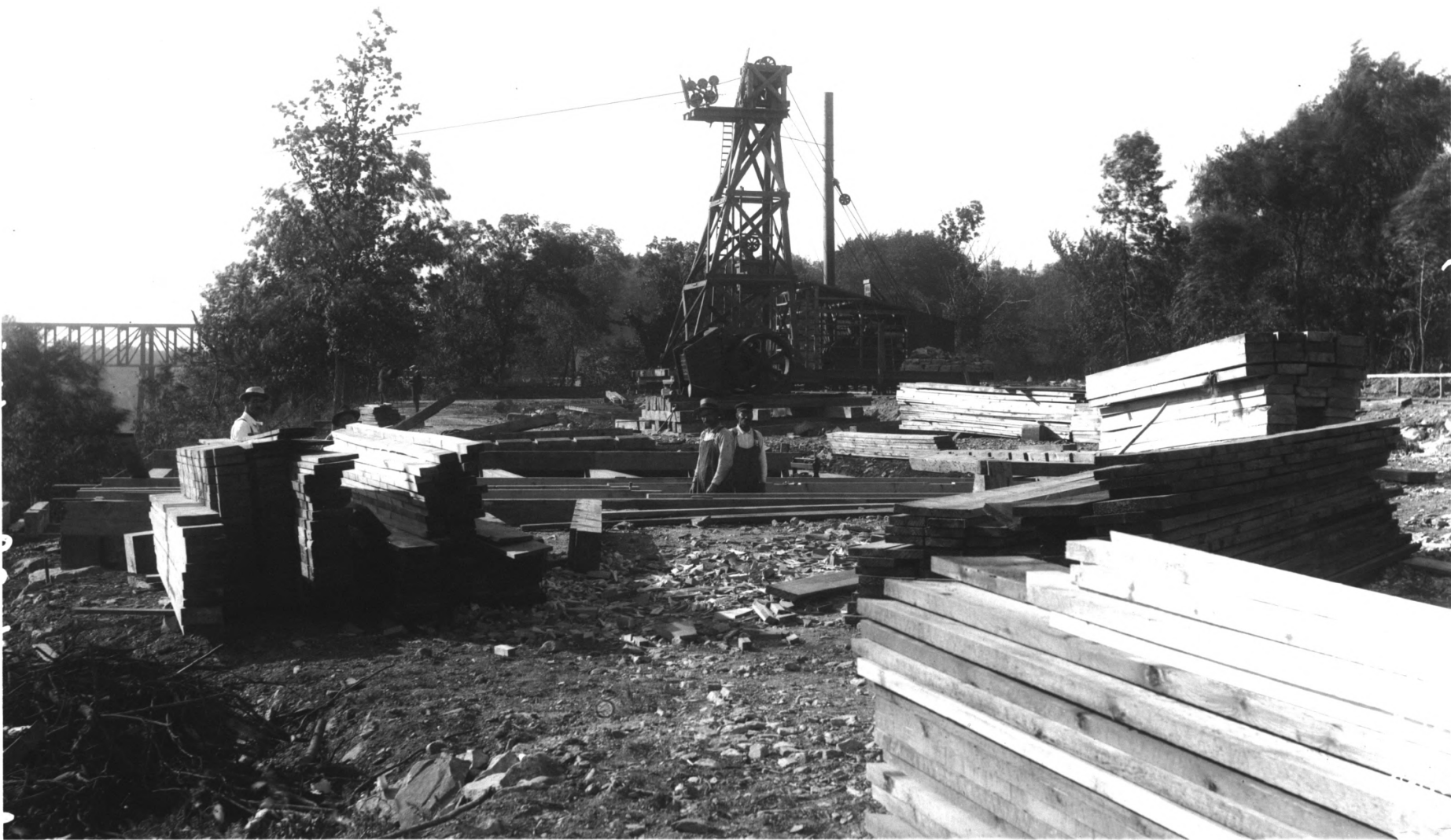
Lock and Dam No. 2 Hennepin and Ramsey Counties, Minnesota MHS 6972A
