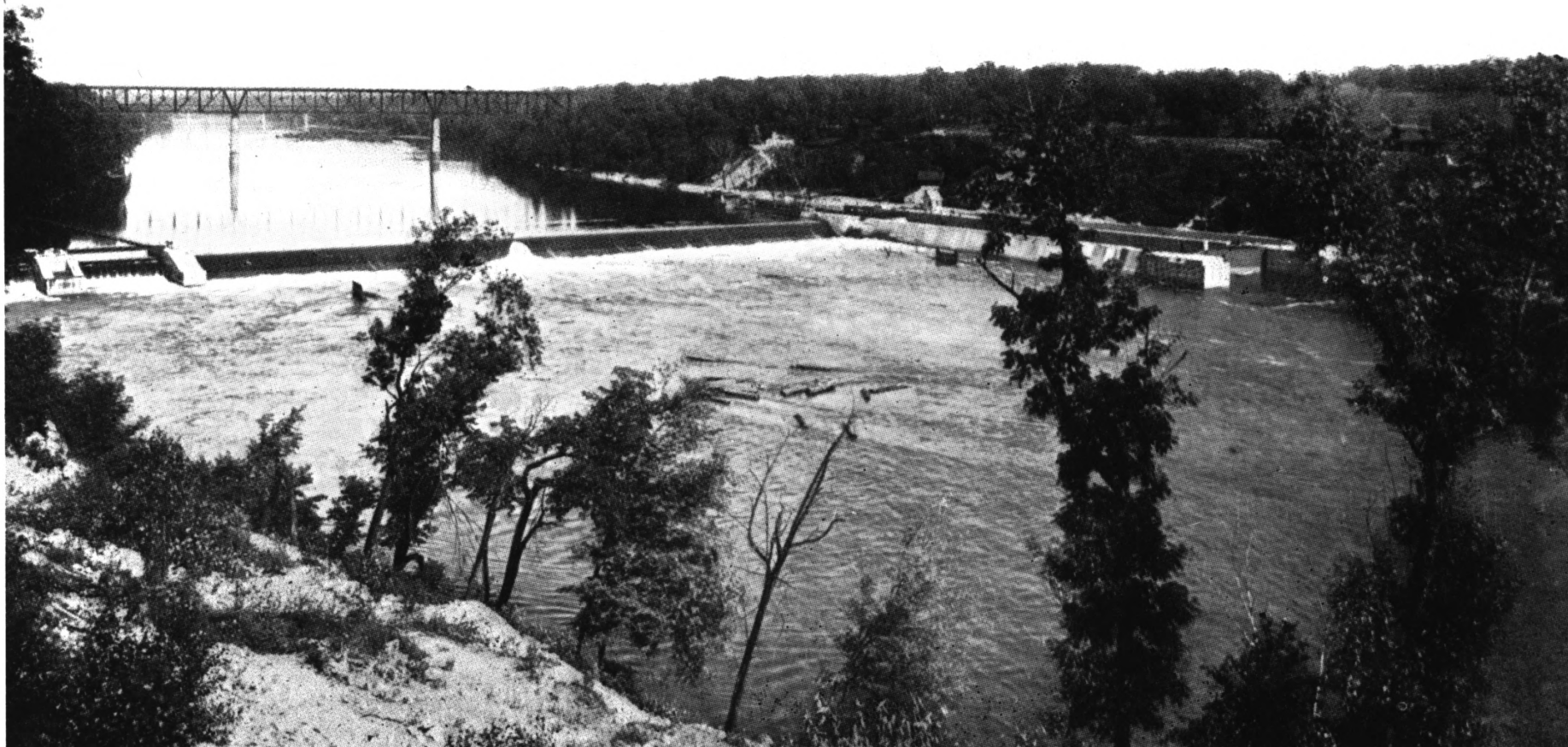
Lock and Dam No. 2 Hennepin and Ramsey Counties, Minnesota MHS 92899
