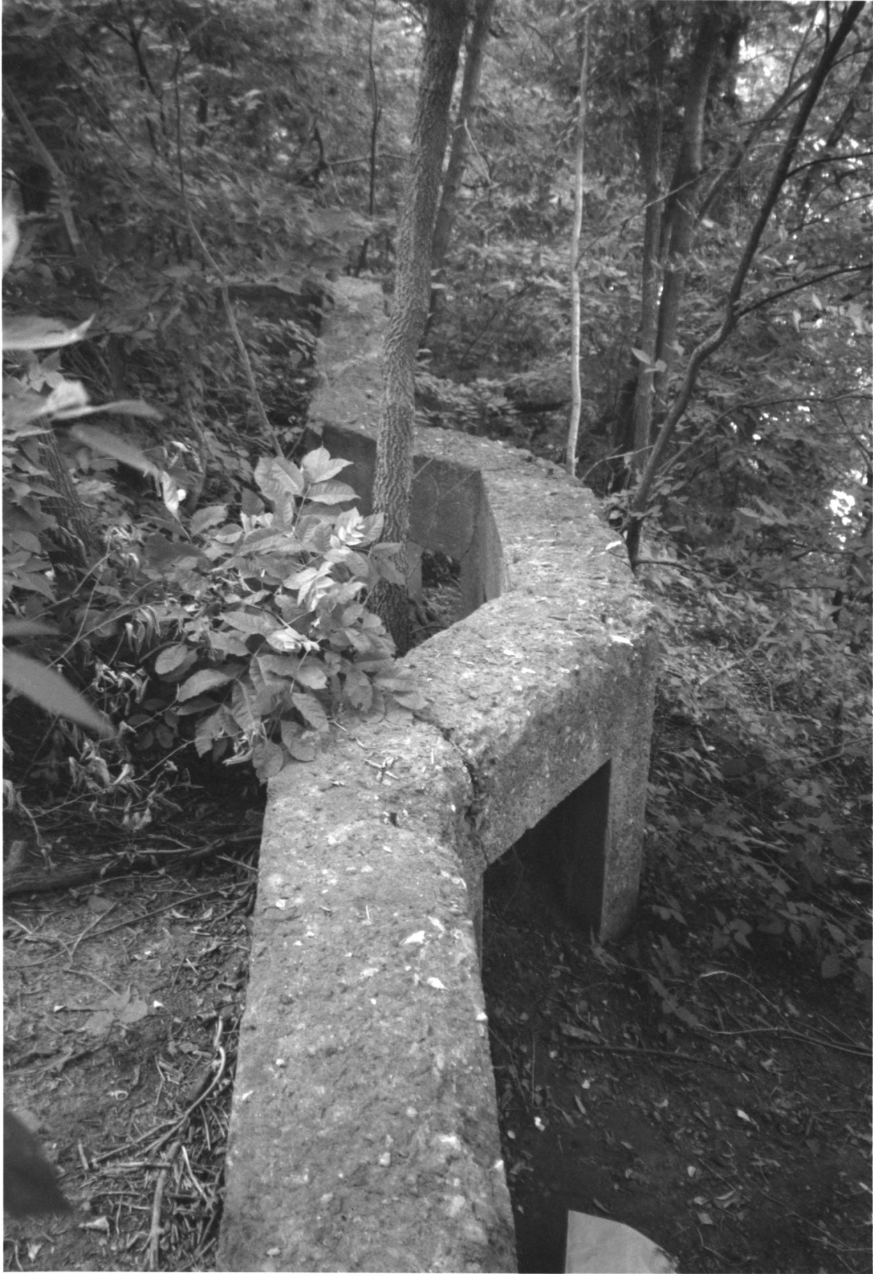
Lock and Dam No. 2 Hennepin and Ramsey Counties, Minnesota MHS 014227-1
