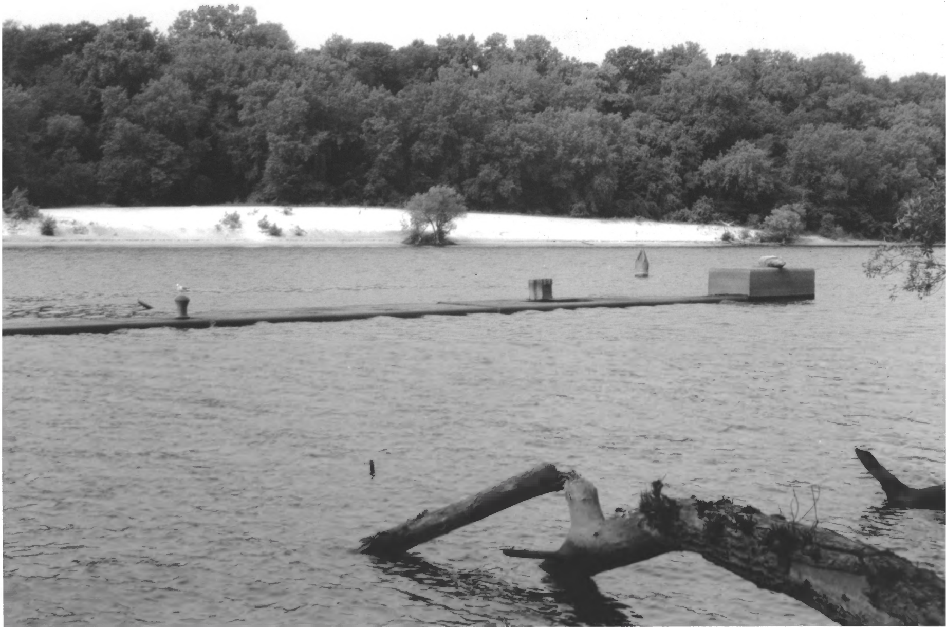
Lock and Dam No. 2 Hennepin and Ramsey Counties, Minnesota MHS 014227-13
