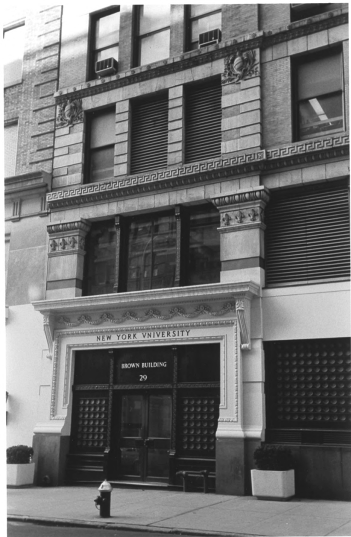
TRIANGLE SHIRTTWAIST FACTORY BUILDING (Brown Building) 23-29 Washington Place, New York, New York Closeup of Entrance Photo by Andrew S. Dolkart, September 1989
