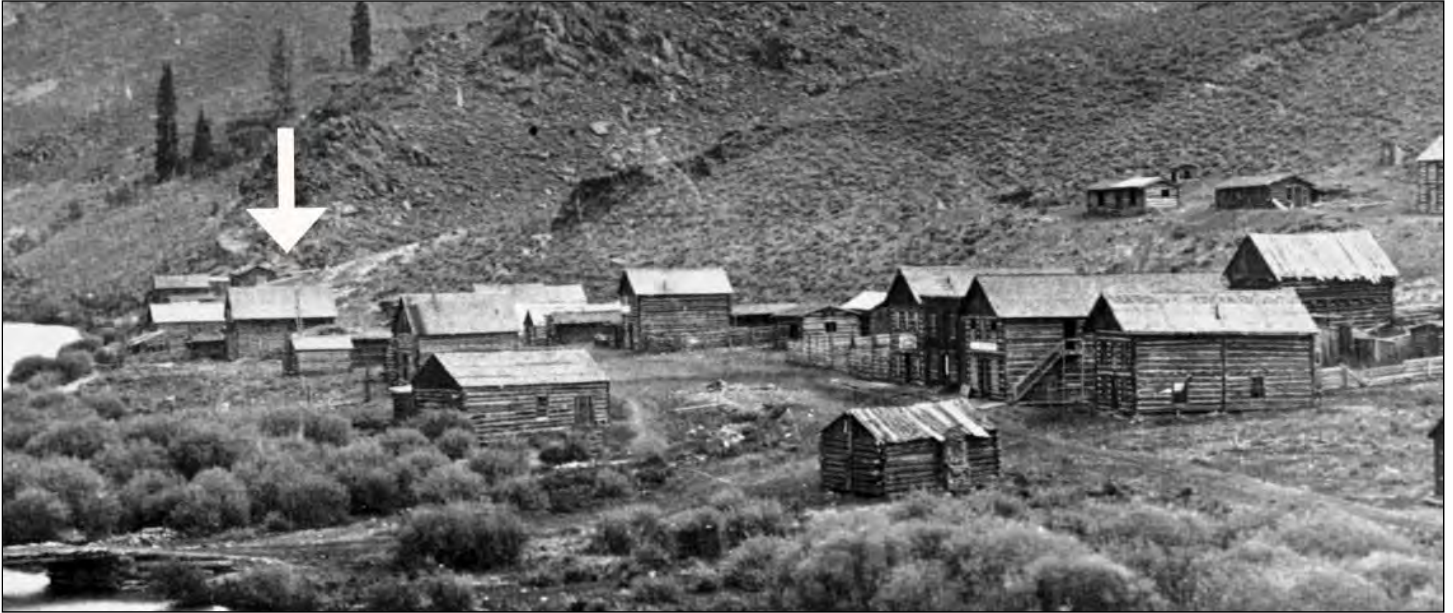
Figure 1. One of the earliest photographs of Granite (ca. 1864-77, view north-northeast) shows the town's log construction without false fronts. The hotel building (arrow) appears, without its north-south wing or rear one-story shed roof addition. The livery stable may be the log building to the north (left and back from the hotel). The photograph predates the 1880 arrival of the D&RG Railroad. Courtesy Denver Public Library, Denver, Colorado, image X-8753.
