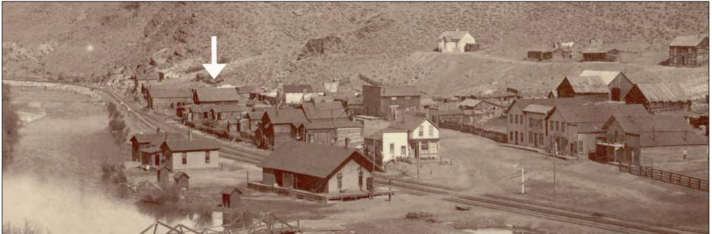
Figure 5. The one-and-a-half-story east-west gabled roof portion of the hotel (arrow) and the one-story shed roof rear section are shown in this image (view north-northeast). Enlargement and examination of this 1890-95 image reveals vertical board-and-batten siding on the south wall. The north-south wing is not present. The log building to the north of the hotel appears to be present beyond and to the left of the hotel; if so, it seems to have a false front on the east. The railroad tracks in the picture have a third rail to accommodate standard gauge cars. The Denver & Rio Grande Railroad made this upgrade in 1890, suggesting the photograph dates to between 1890 and 1895, when the north-south section is shown in a photograph (see Figure 6). Courtesy of History Colorado, Denver, Colorado, image X-4937.
