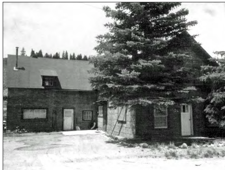
Figure 9. The hotel building was clad with rolled asphalt siding resembling brick in 1974 (view west-northwest). Courtesy of History Colorado, survey form photograph, 5CF.155, 1974.
