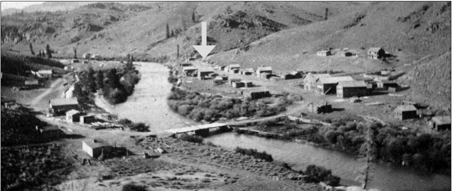
Figure 2. This view northeast of Granite shows the hotel building (arrow). The photograph appears in Digerness, The Mineral Belt , vol. 1, 236, with an attributed date of 1876. Courtesy of Western History and Genealogy Department, Denver Public Library, Denver, Colorado, W.G. Chamberlain photograph, image number X-8752.
