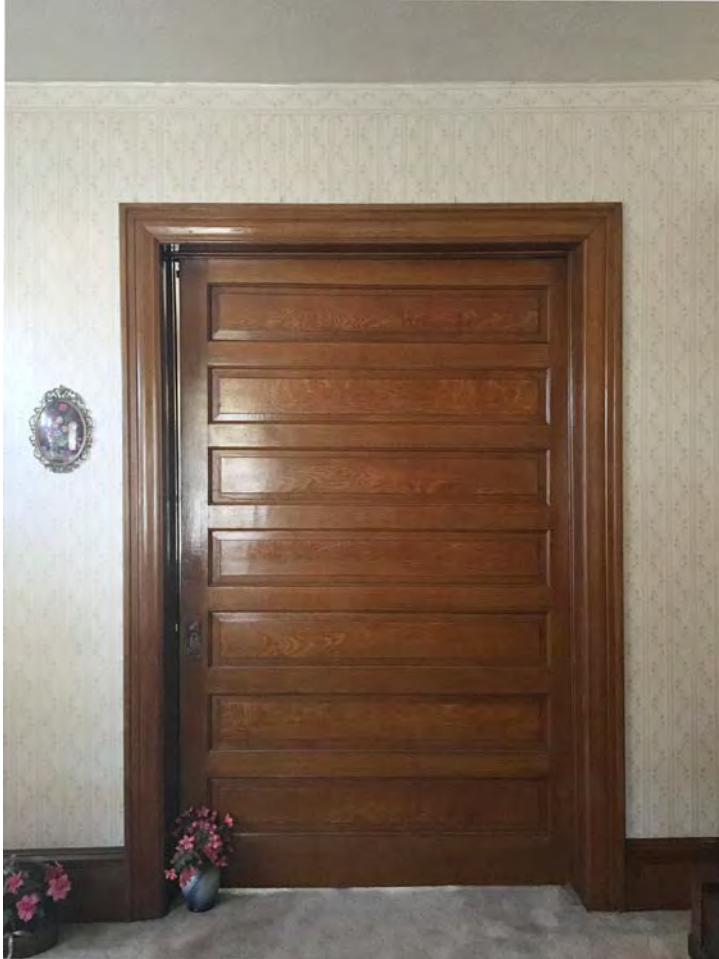
Photo 11. Date: 11/13/2016. Description: Interior, faux hardwood-painted pocket door. Camera facing south.
