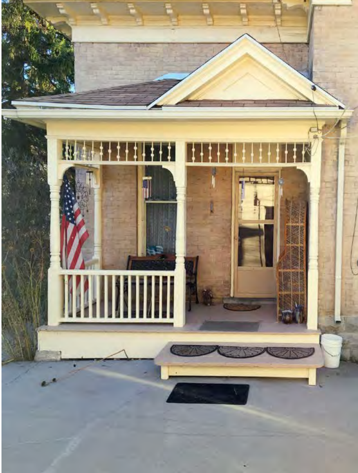
Photo 5. Date: 11/13/2016. Description: North porch, camera facing south.
