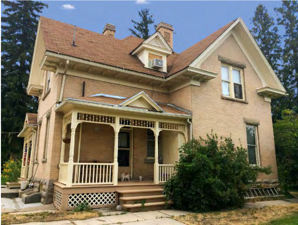
Photo 3. Date: 8/25/2016. Description: West elevation, camera facing east.
