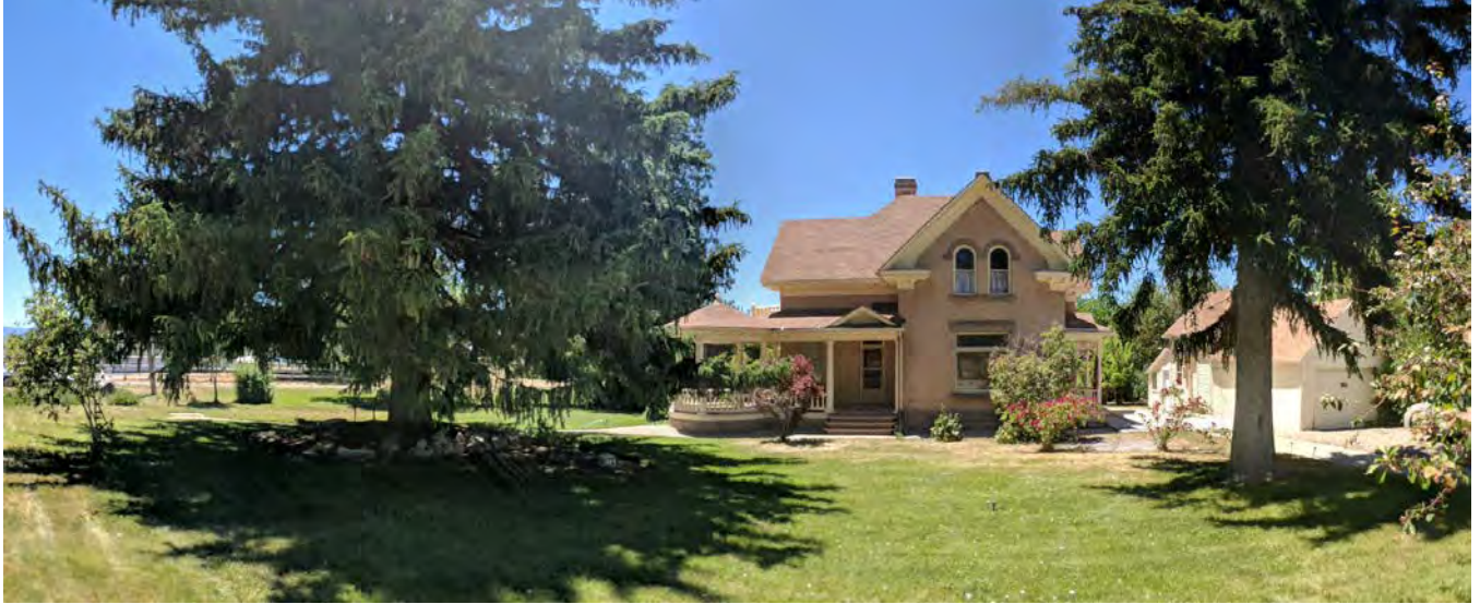
Photo 6. Date: 6/25/2018. Description: East yard, house, garage, washhouse, coal shed. Camera facing west.
