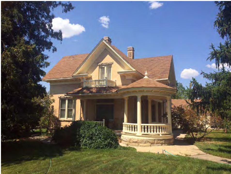
Photo 2. Date: 8/18/2016. Description: South elevation of the house, camera facing north.
