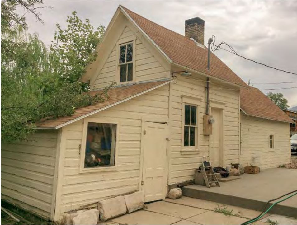
Photo 12. Date: 6/25/2018. Description: Coal shed (left), washhouse (middle), garage (right). Camera facing northeast.
