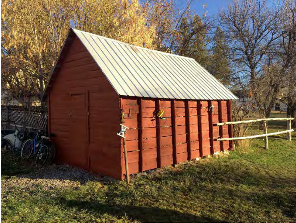
Photo 15. Date: 11/13/2016. Description: Granary, camera facing southeast.
