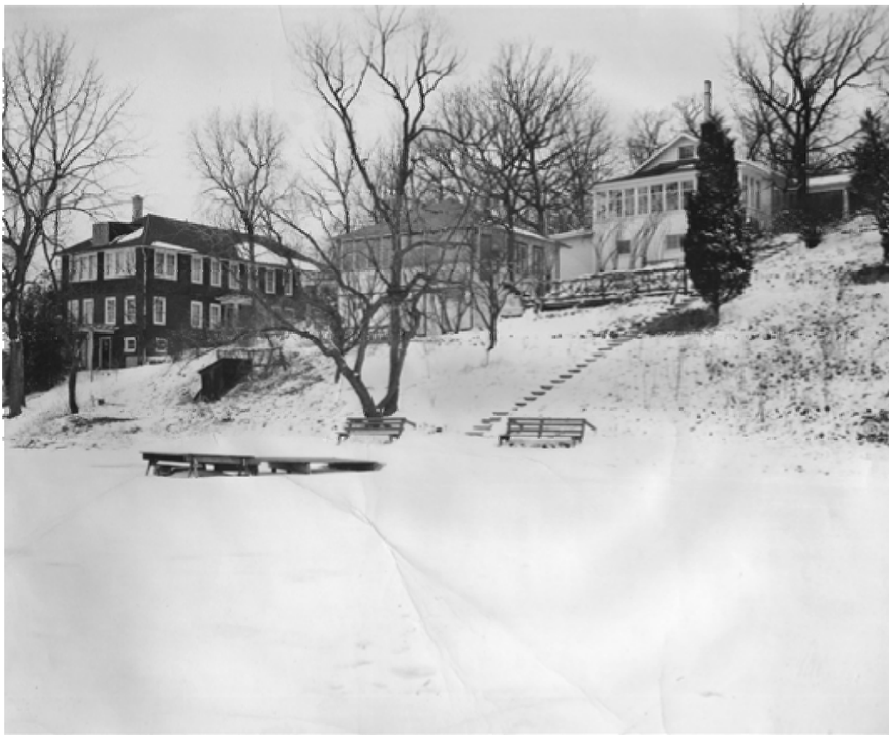
Wandawega Lake Resort - Hotel, 3-Bedroom Cabin & Lodge, c. late 1940s – 1950s
