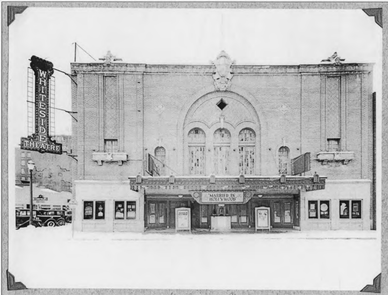
Front facade of the Whiteside Theatre in c.1930. Courtesy of Benton County Historical Society & Museum.
