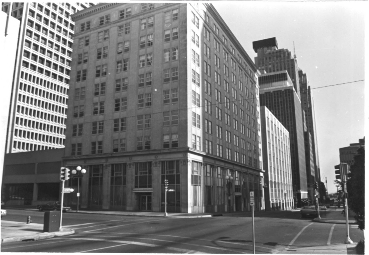
EXHIBIT G - THREE TWENTY FOUR BUILDING (1980)
