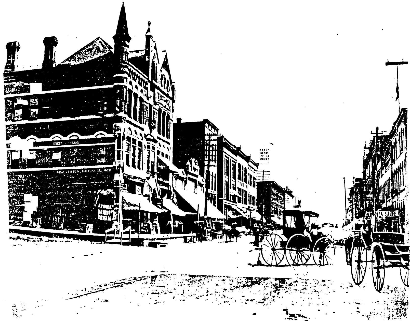
corner of 5th & Jefferson, view to the northeast
