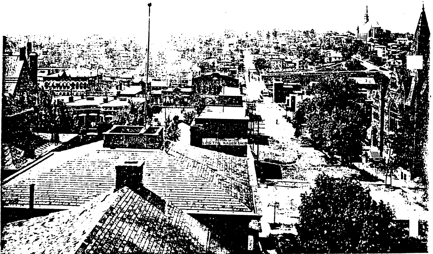
view to Jefferson Street from 6th & Columbia Mozart Hall (#140) in center from 1889 Burlington Illustrated on file Burlington Public Library
