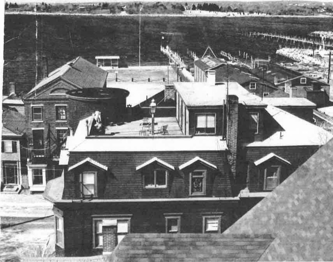
Archival Image 3: Merrill House with rooftop addition and deck, looking west
