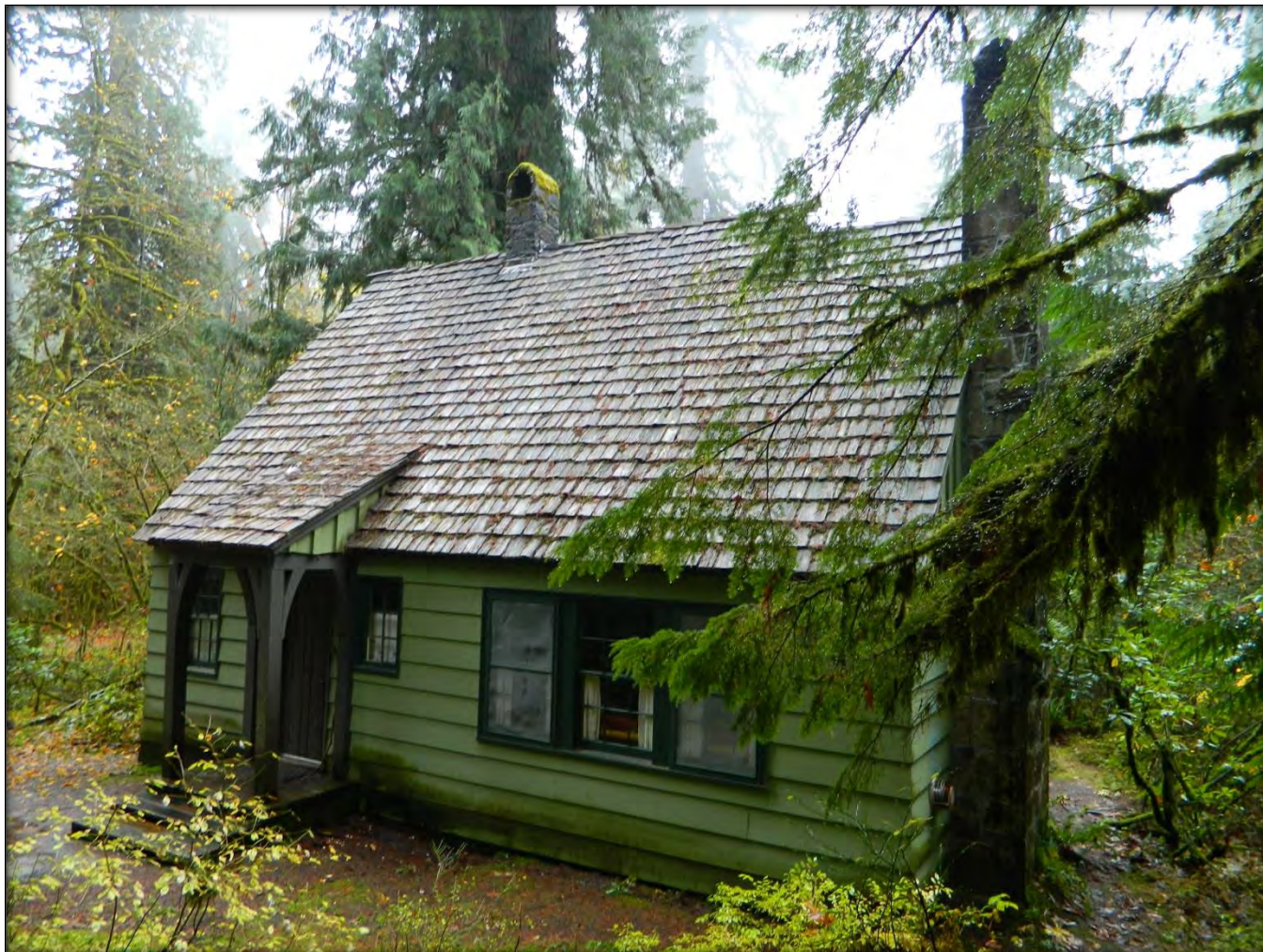
Photograph #5 - Southwest elevation with back porch, exterior chimney (on right), and interior chimney (center top). Photo taken at an angle due to vegetation obstructing a clear perpendicular shot
