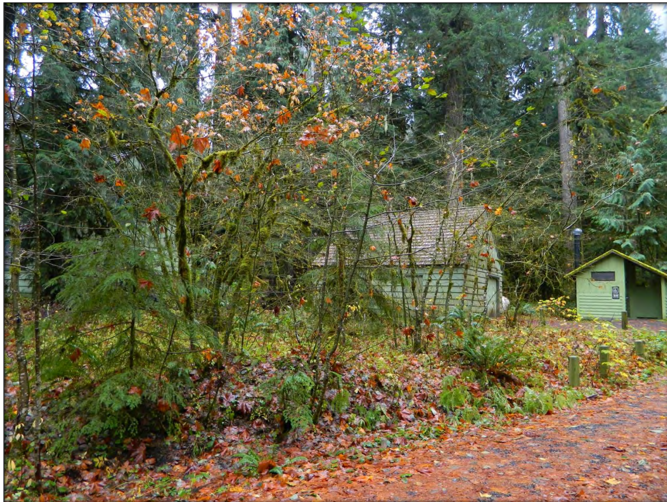
Photograph #10 - Photograph showing the spatial relationship of the GMS Guard Station (midground left partially obscured by vegetation), the garage, midground center) and the modern vault toilet (midground right)
