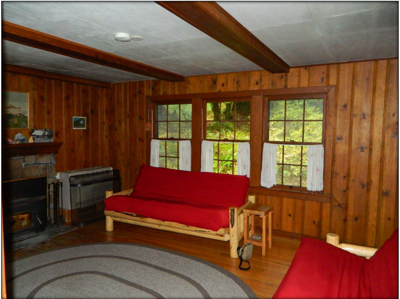
Photograph #12 - Living room taken from primary entrance to the structure showing triple six-over-six wood sash windows with mullions
