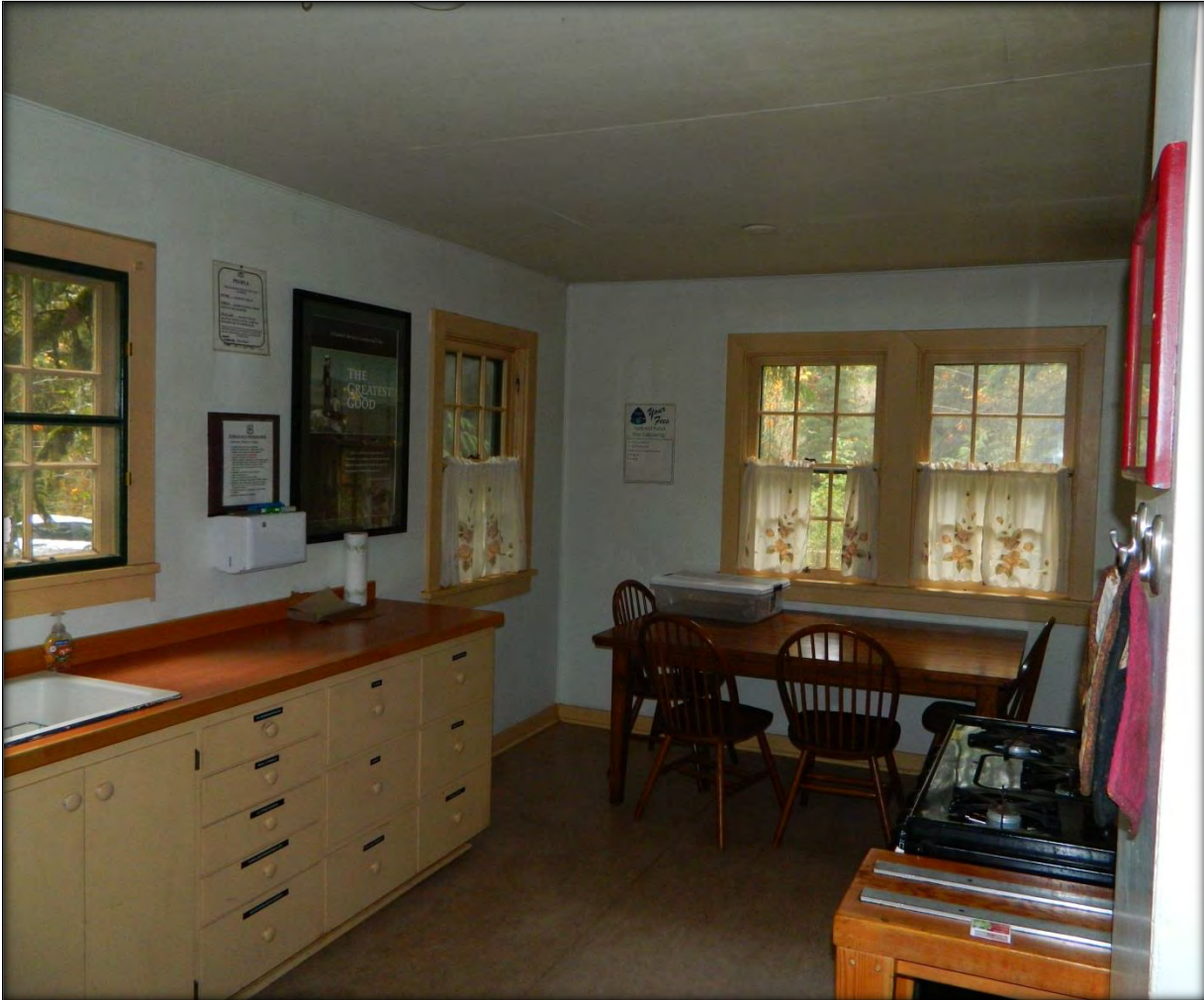
Photograph #16 - Kitchen with table and chairs, range (right) with sink and cupboards (left). Also shown are double six-over-six wood sash windows with mullion above table, single six-over-six wood sash window to left of table, and portion of six-over-six wood sash window above sink
