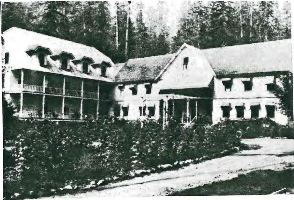
Photograph #31 - 1920 Photo of the Government Mineral Springs Hotel with addition and some alterations to the front façade
