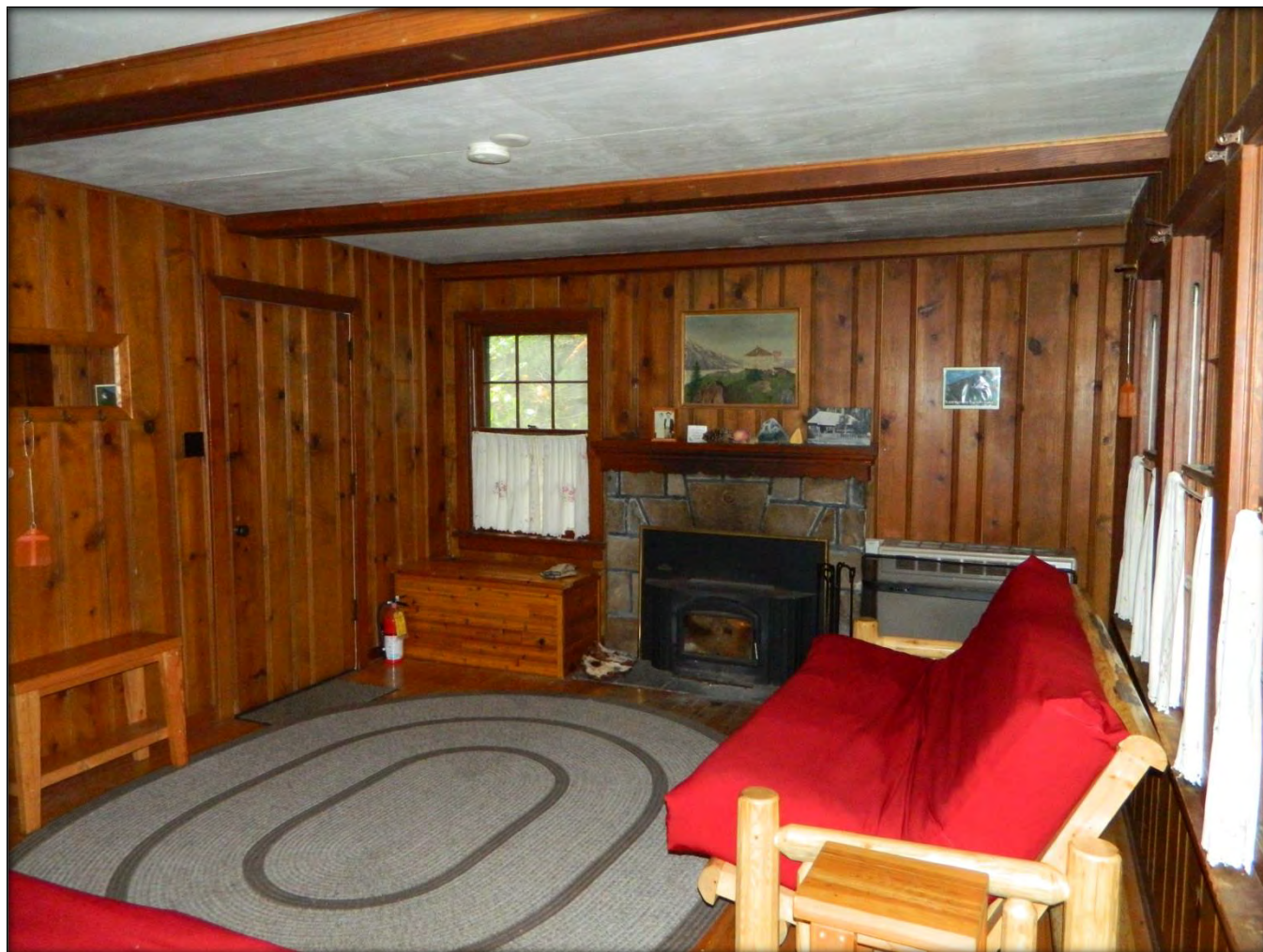
Photograph #11 - Living room with fireplace, knotty pine paneling, four six-over-six wood sash windows, 4"x8" trimmed pine open beams on the ceiling, and furniture
