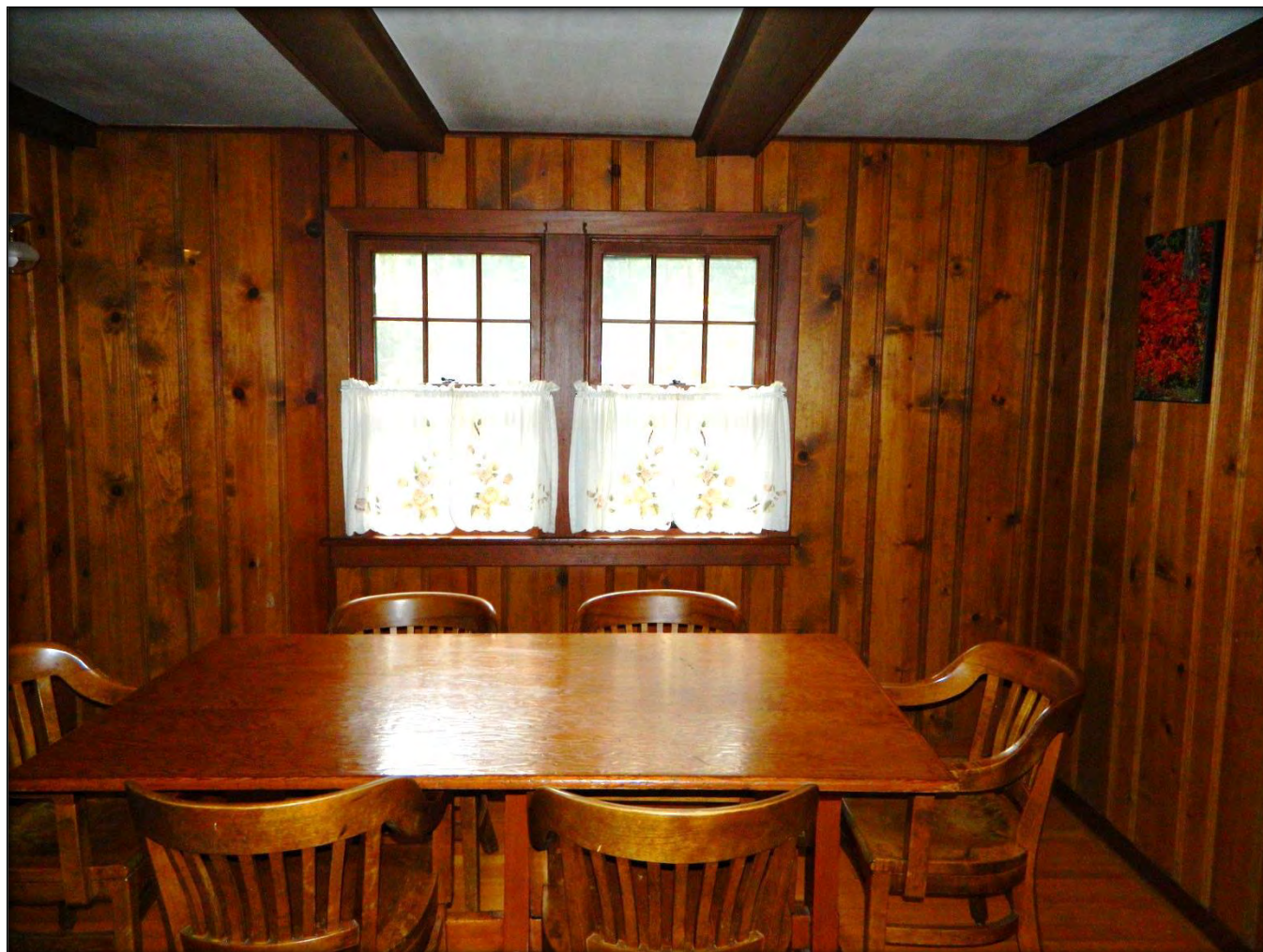
Photograph #15 - Dining room/office with table, chairs, and double six-over-six wood sash windows with mullion
