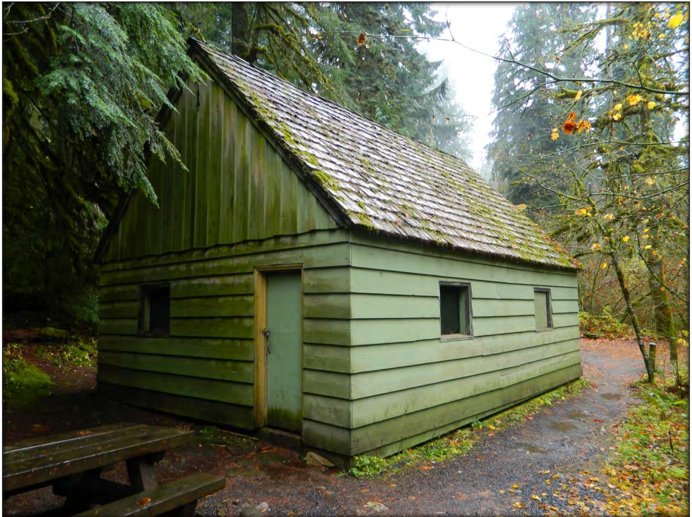
Photograph #8 - Garage - Side and back elevations
