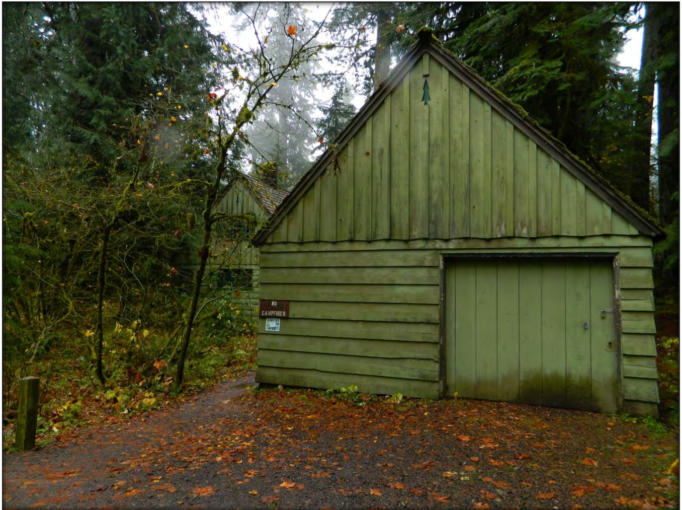
Photograph #7 - Garage - Front (NW) elevation with Guard station in background (left)
