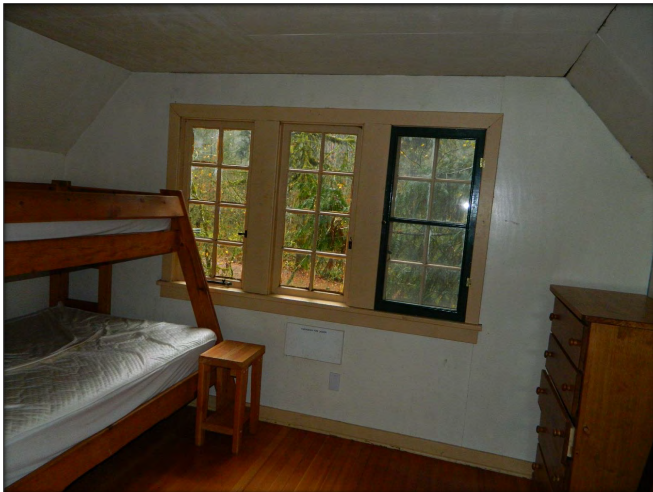
Photograph #25 - Second bedroom with bunkbed, dresser, nightstand, and triple eight-pane casement wood windows with mullions and screen on right window
