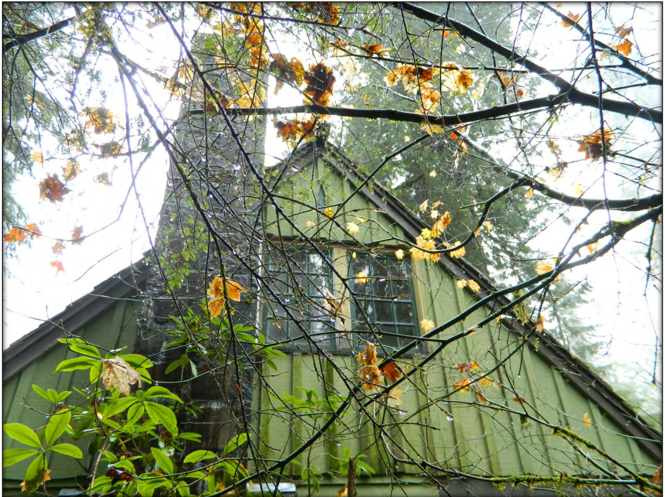
Photograph #4 - Gable portion of southeast elevation
