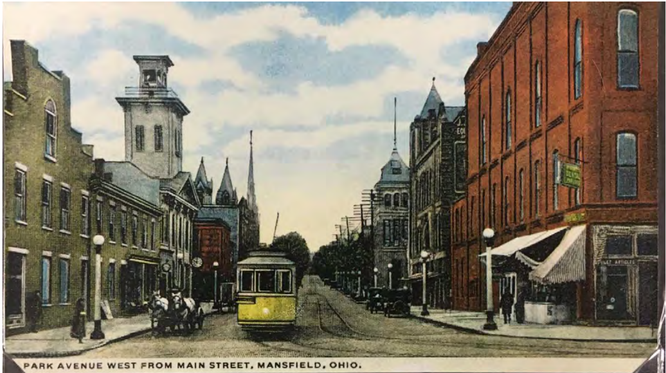
Illustration 7: A colored illustration of the electric streetcar line on Park Avenue West as seen from North Main Street. This line was one of the first services of its kind in the state of Ohio.
