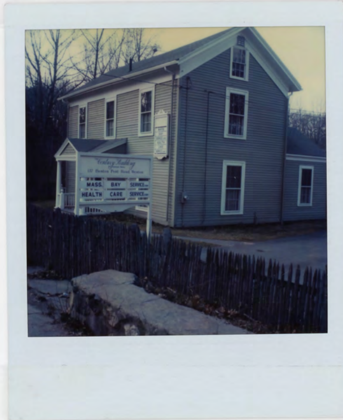
137 Boston Post Road - Large free-standing advertising sign and sign on structure dominate front yard of property. Large paved parking lot on easterly side of property is visible to the right of the office building.
