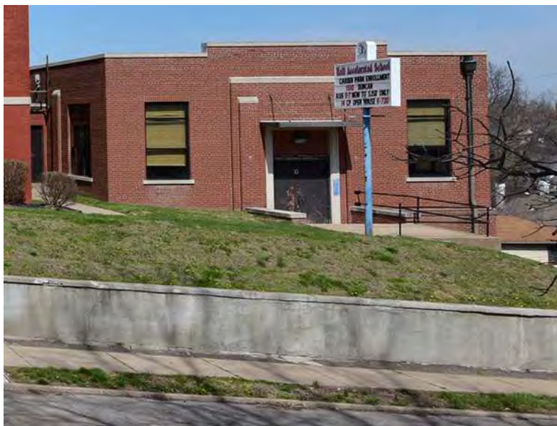
Figure 14. Hall School Block C, south elevation. Source: Brad Finch, 2016.
