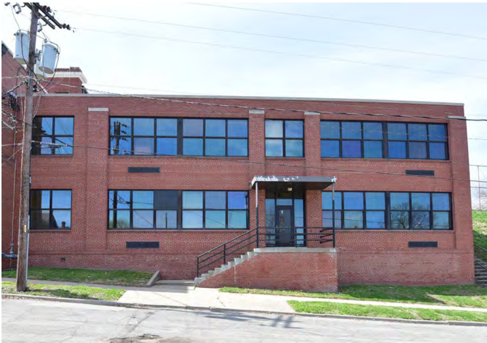
Figure 15. Hall School Block E, east elevation. Source: Brad Finch, 2016.
