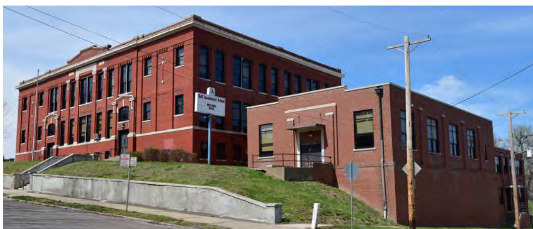
Figure 11. Hall School Main Block, south and east elevations. Source: Brad Finch, 2016.
