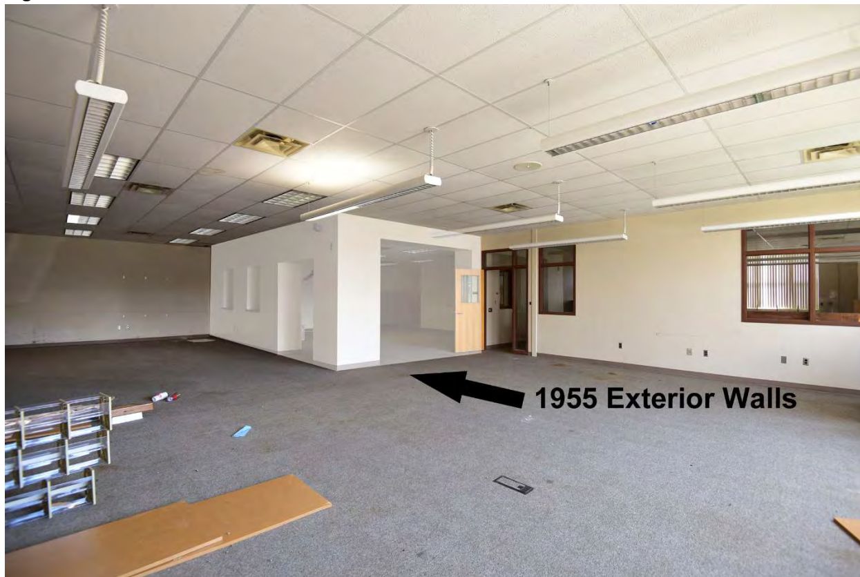
Figure 24. Exterior walls of 1955 addition in the 2001 addition. Source: Brad Finch, 2016.
