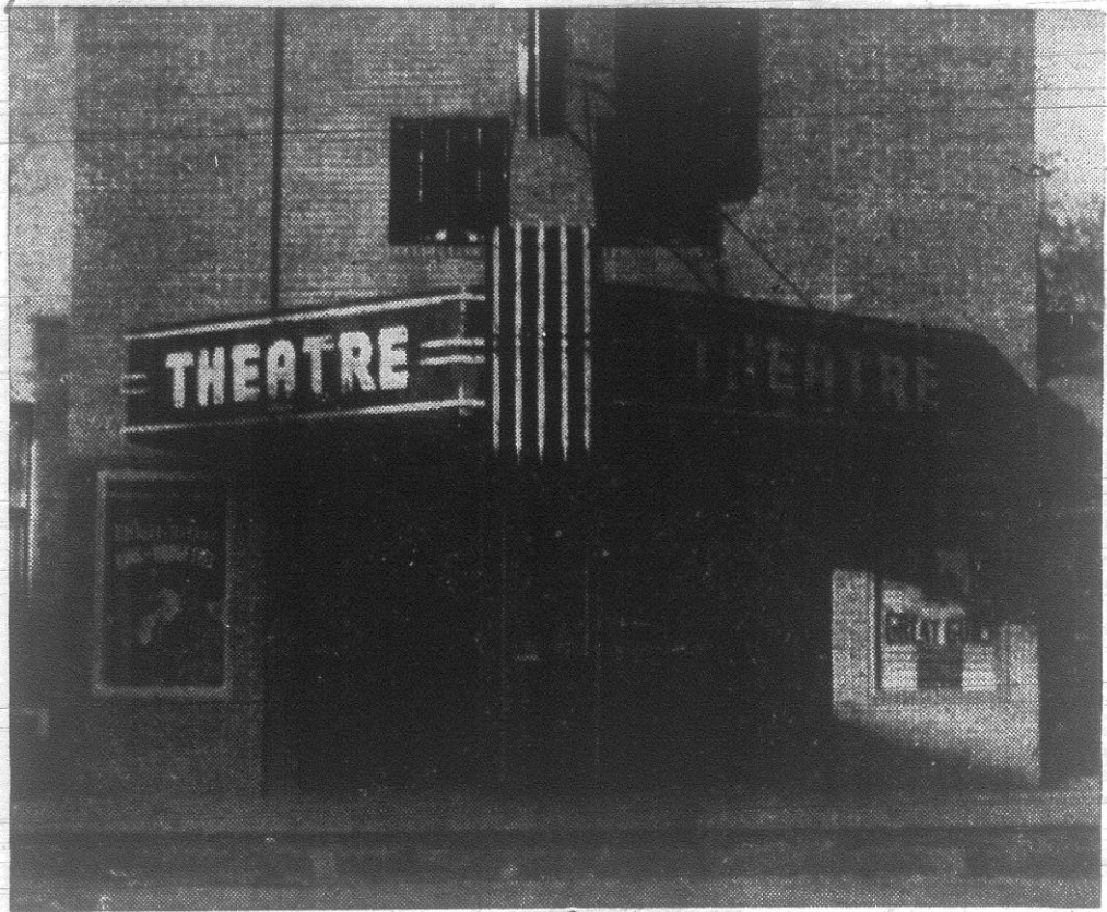
New Theatre Façade (South Elevation) November 1941
