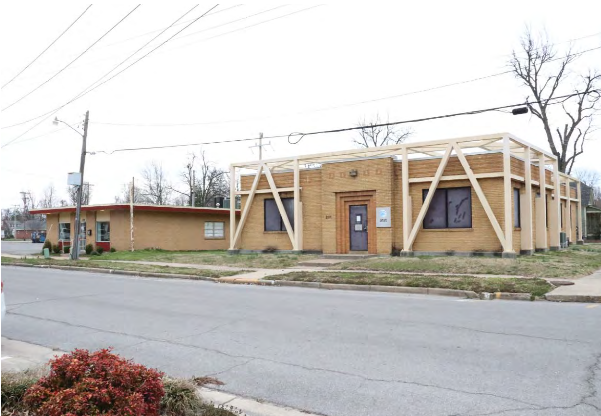
One Part Commercial Block Postwar Art Deco, 201 North 1st Street Visible from the North Elevation of the McCutchen Theatre
