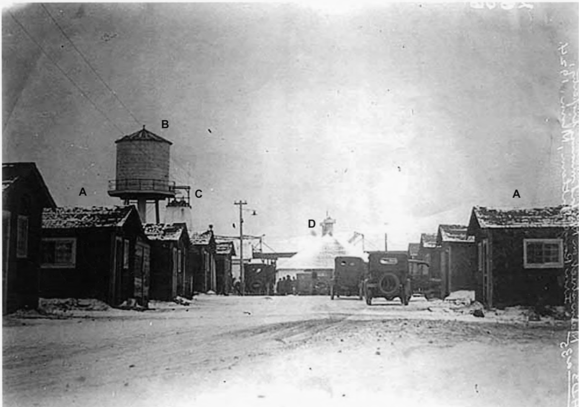
Main Street of the Milford Mine Complex, 1924, view to north. (A: Miners' Housing; B: Water Tower; C: Headframe; D: Dry House)
