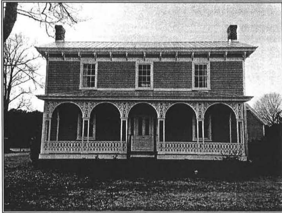
Figure 1. Pugh House, east facade.
