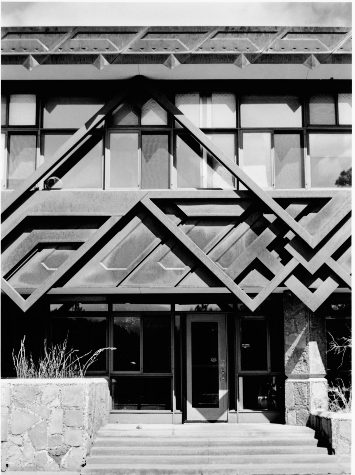
Figure 3 Rocky Mountain National Park Administration Building Larimer County, Colorado Staff entrance, 1999
