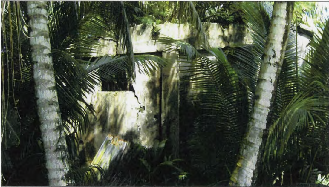
Figure 18. Exterior of west side of the building.
