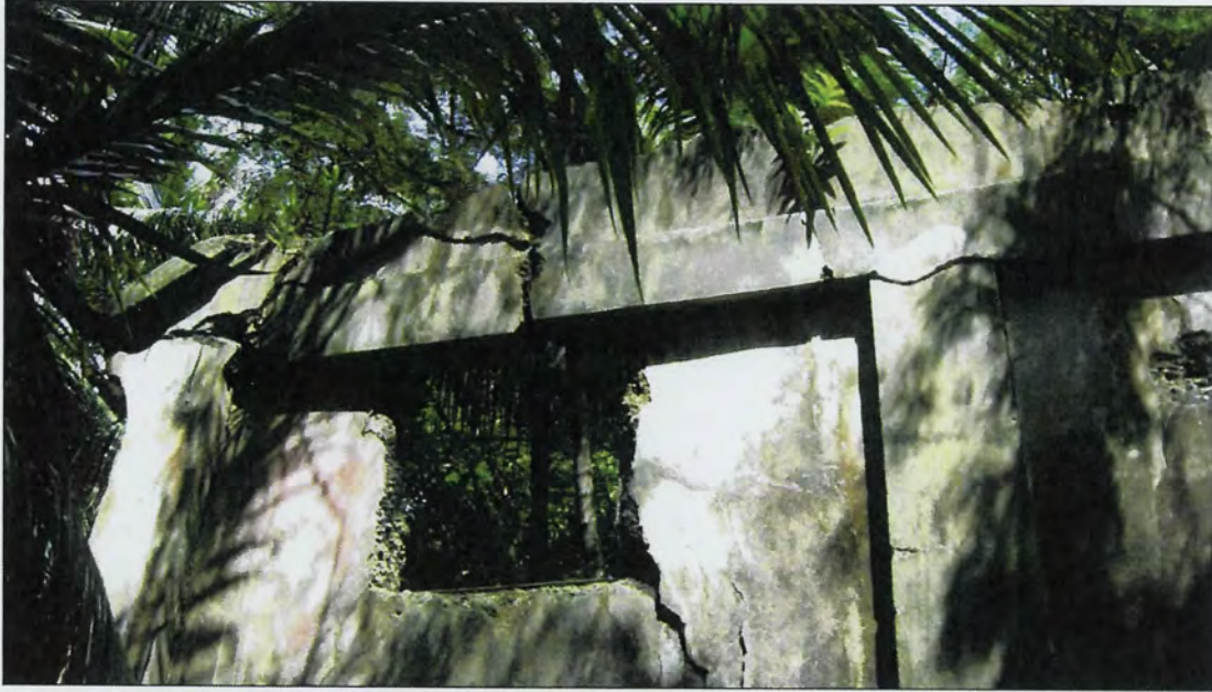
Figure A-10. Northern window on the west side of the building.
