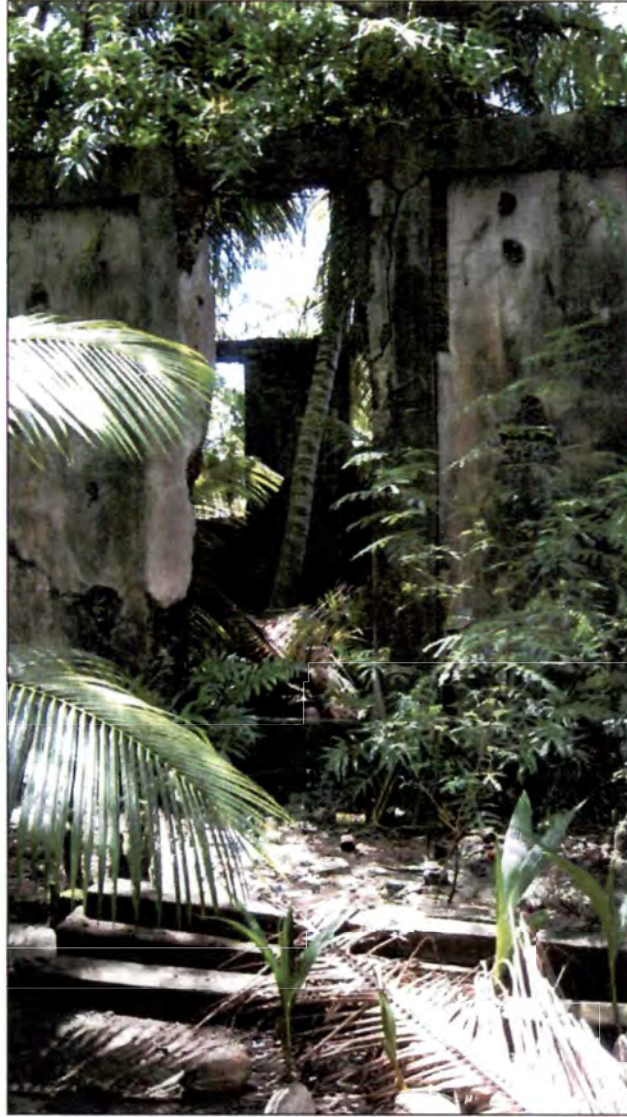
Figure 16. Eastern entrance on the north side of the building.
