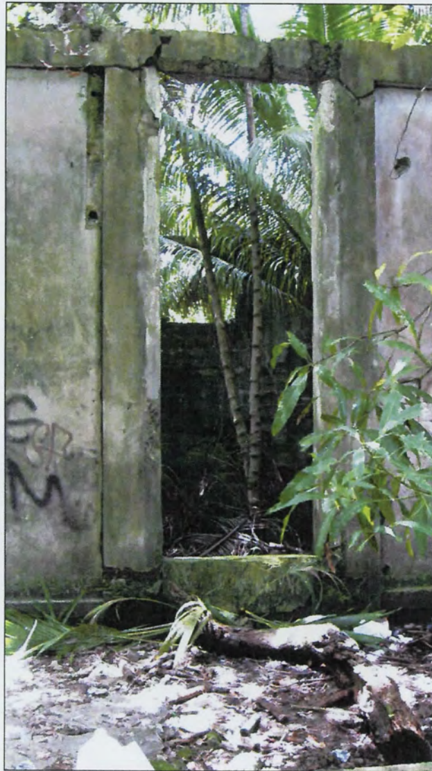
Figure A-6. Western entrance on the north side of the building.
