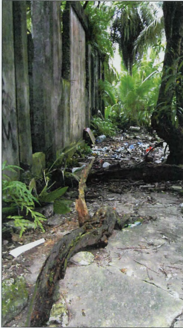
Figure A-15. Concrete slab facing west.
