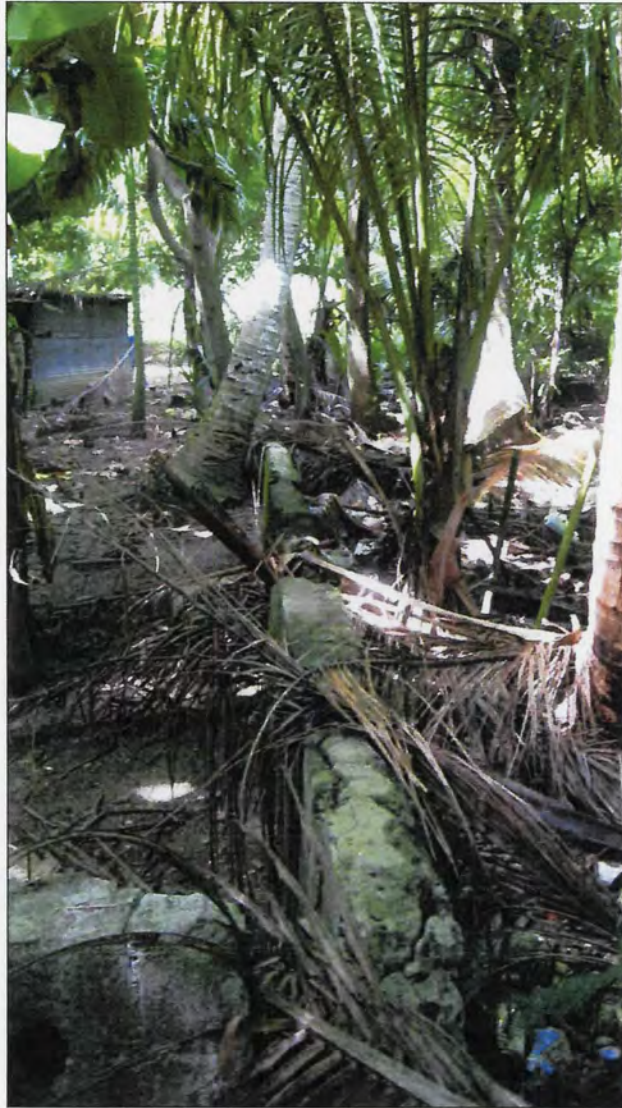
Figure 23. Low retaining wall running north onto neighboring property.
