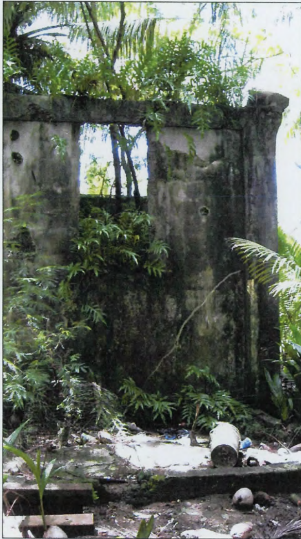
Figure A-7. Eastern most window of the north wall.
