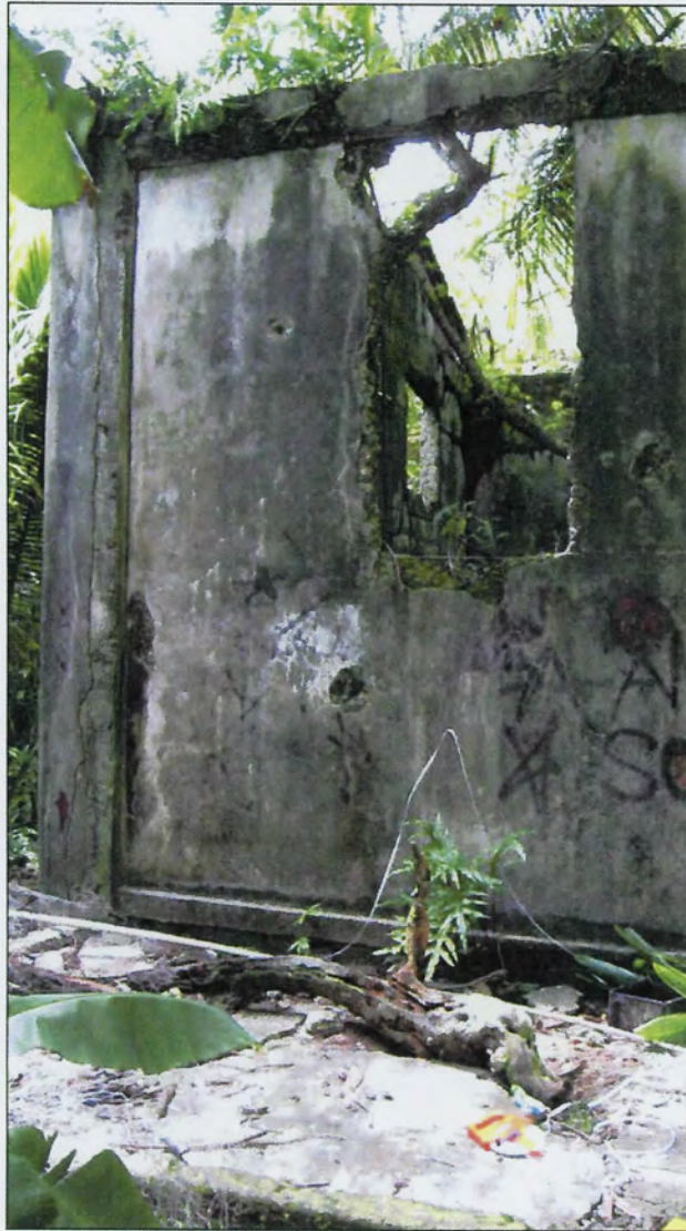
Figure A-9. Westernmost window of the north wall.
