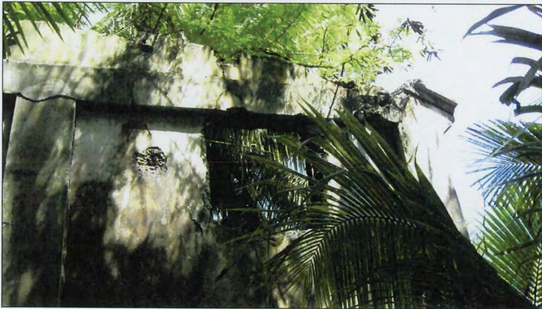
Figure A-11. Southern window on the west side of the building.
