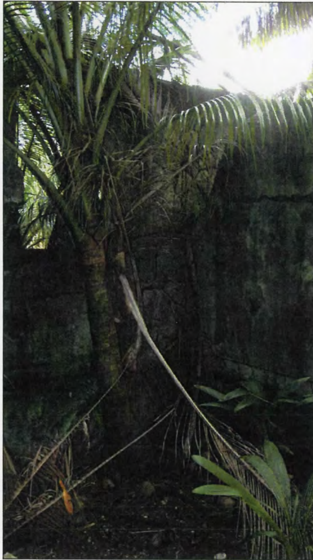
Figure 20. Interior of east room facing southwest.
