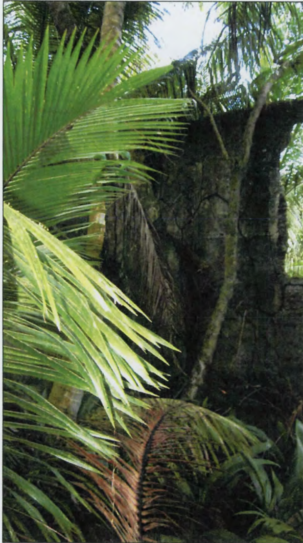
Figure A-14. Interior of west room facing south.
