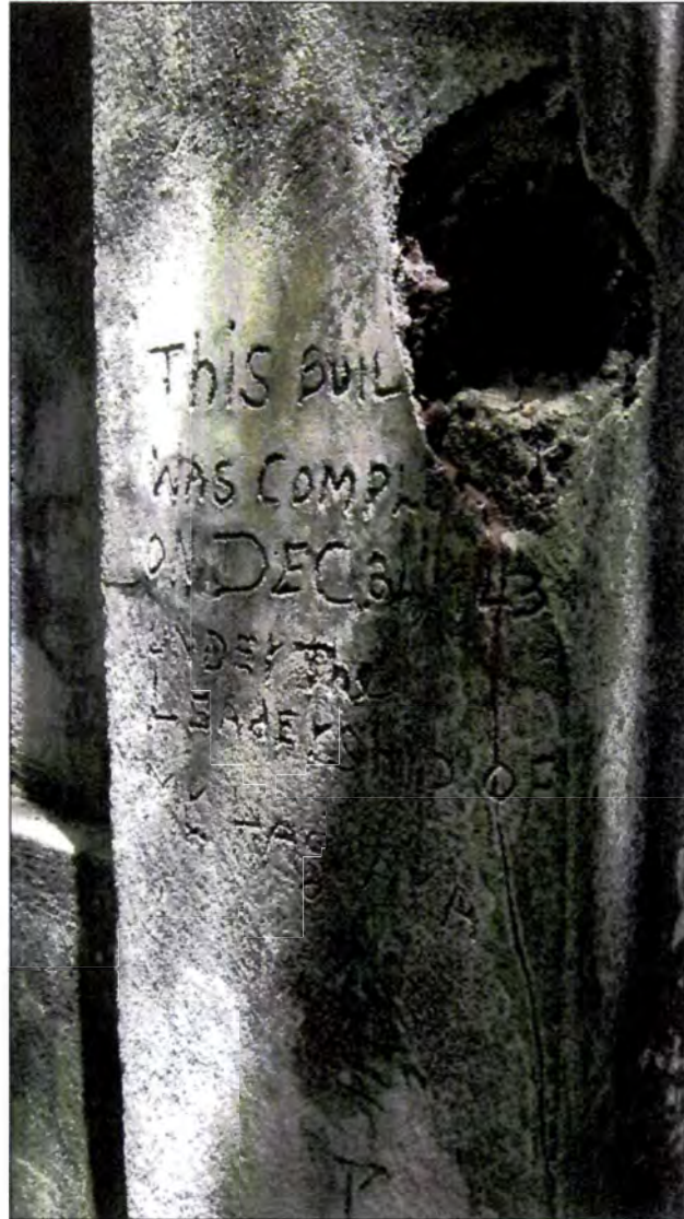
Figure 15. Inscription on southwest corner of the rear wall.
