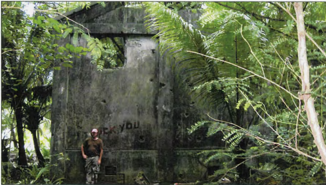
Figure 19. East side of the building. Note vents at the base of the wall.
