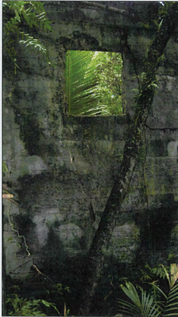
Figure A-12 Interior of east room facing southeast.
