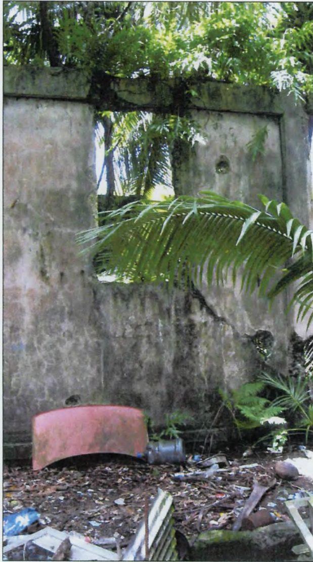
Figure A-8. Middle east window of the north wall.
