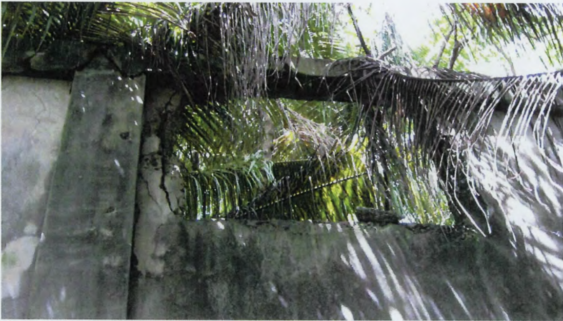
Figure A-3. Easternmost window on south wall.
