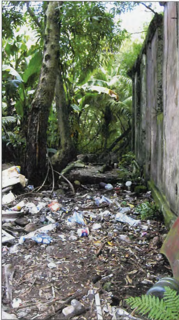
Figure 22. Concrete slab facing east.
