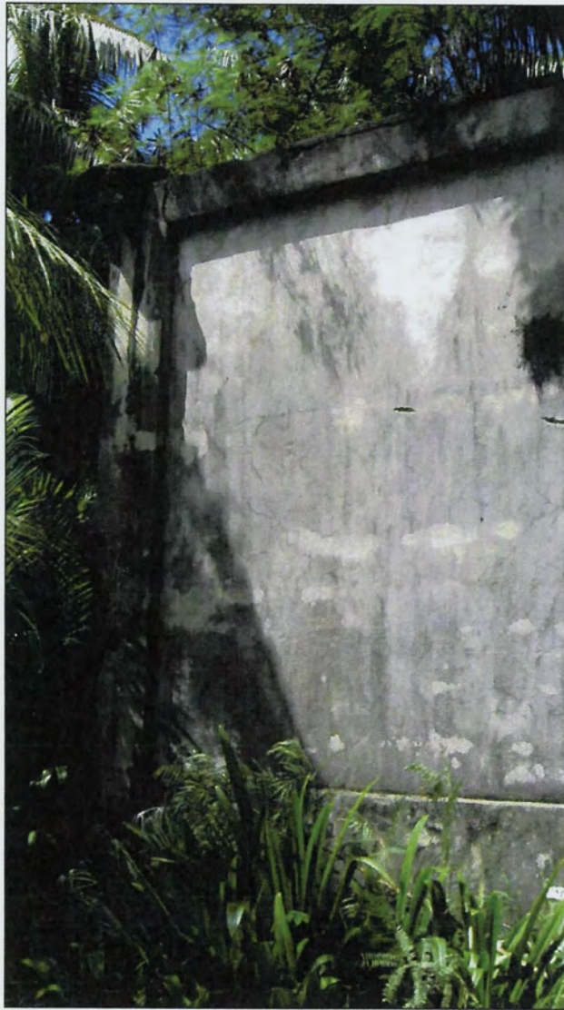
Figure A-2. West corner of south wall.
