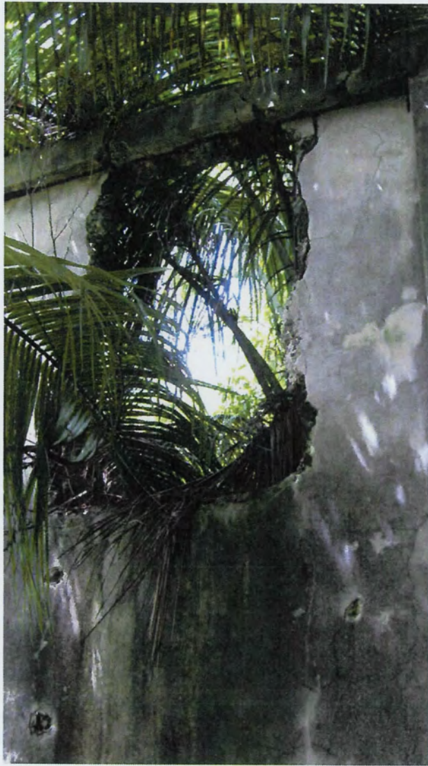
Figure A-5. Middle east window on south wall.
