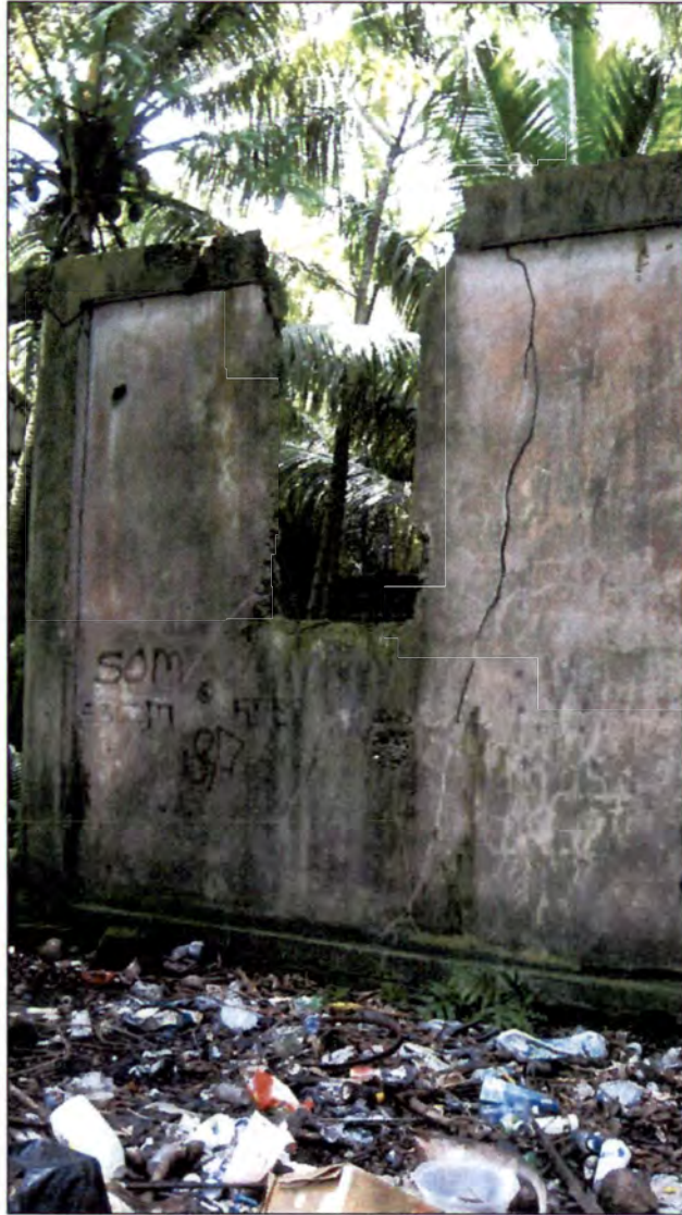
Figure 17. West middle window of the north wall.
