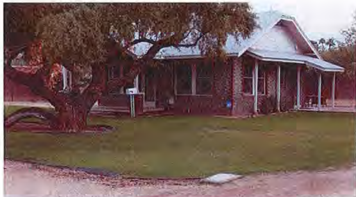
Figure 38. The ca. 1930 bungalow at 341 W. Hazelwood St. was constructed in brick in a side gabled form with front facing gabled porch across about half the façade. This house features decorative quoins in brick at the corners and window openings. Source: Google, 2015.
