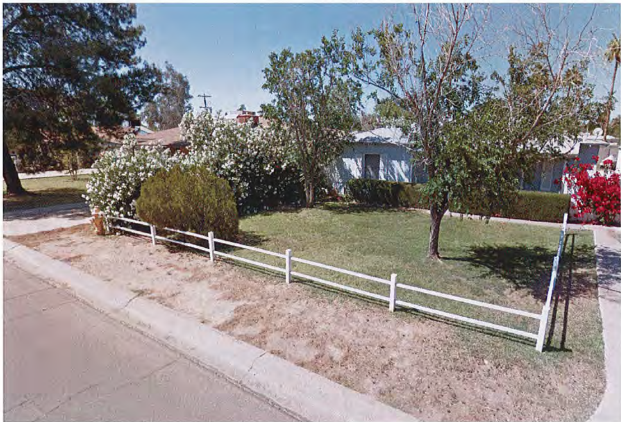
Figure 45. The house at 138 W. Highland Ave. illustrates several features of Pierson Place Historic District's character. It was built in 1947, the district's most active construction year, in the Transitional Ranch form that is the district's primary stylistic aesthetic. Streets are paved with curb and gutter, here rolled, a form more conducive to rapid construction. The district has no sidewalks, a characteristic of its development outside of what was then Phoenix's city limits. Landscaping has been individualized by property owners. Source: Google, 2016.
