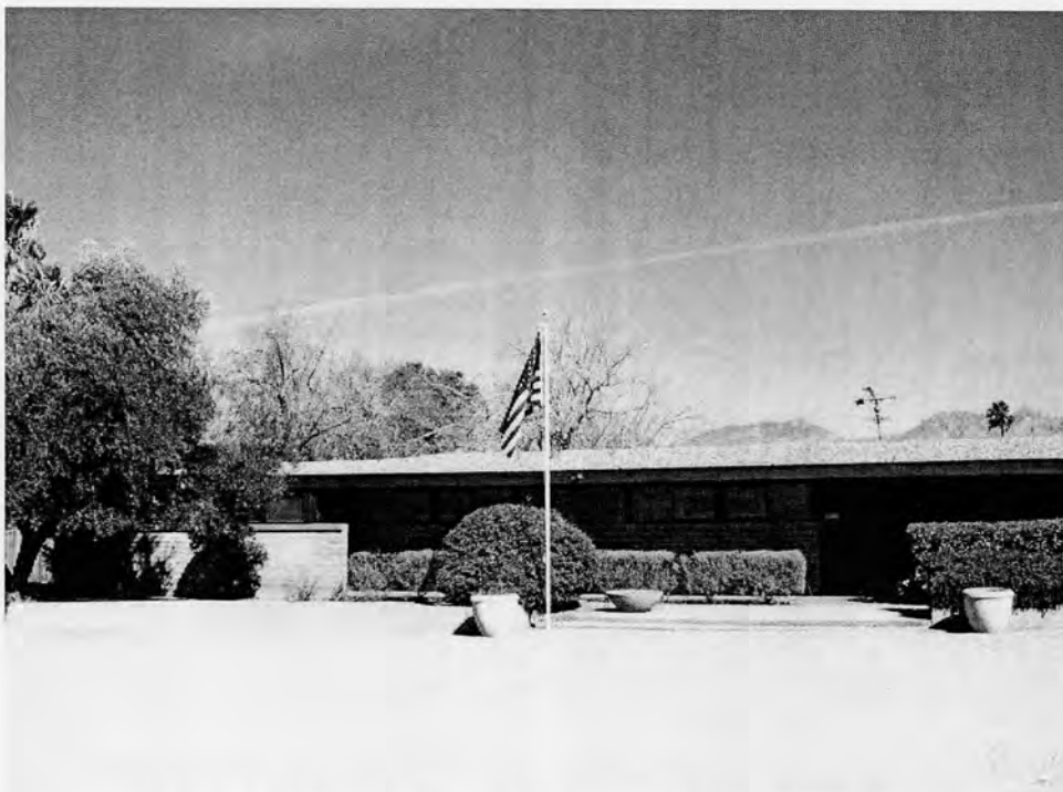
Figure 33. 6425 E. Brian Kent St.; view north-northwest.
