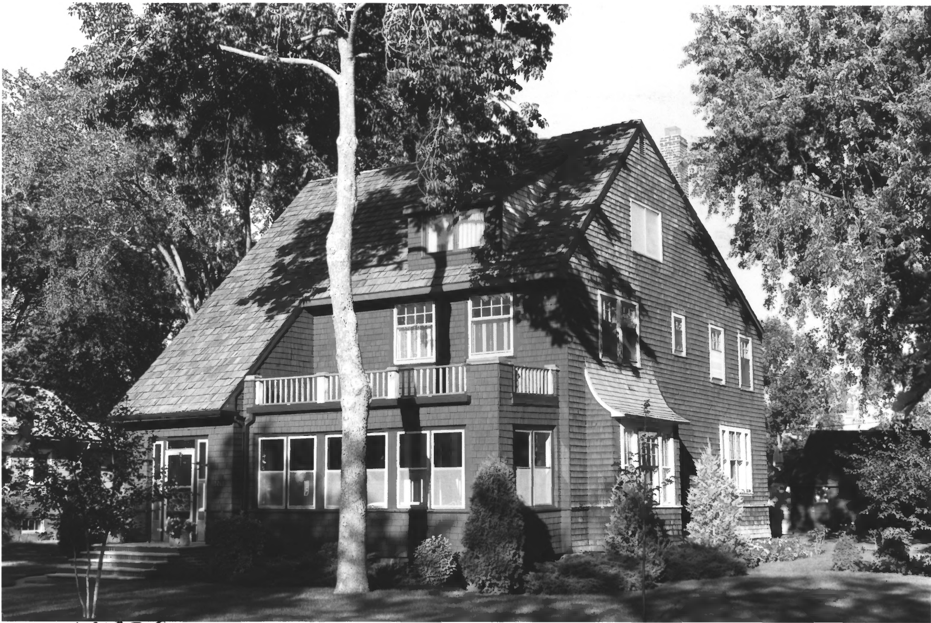
1011 DOUGLAS ST. ALEXANDRIA RESIDENTIAL HISTORIC DISTRICT ALEXANDRIA, DOUGLAS CO., MINNESOTA 010611 #6
