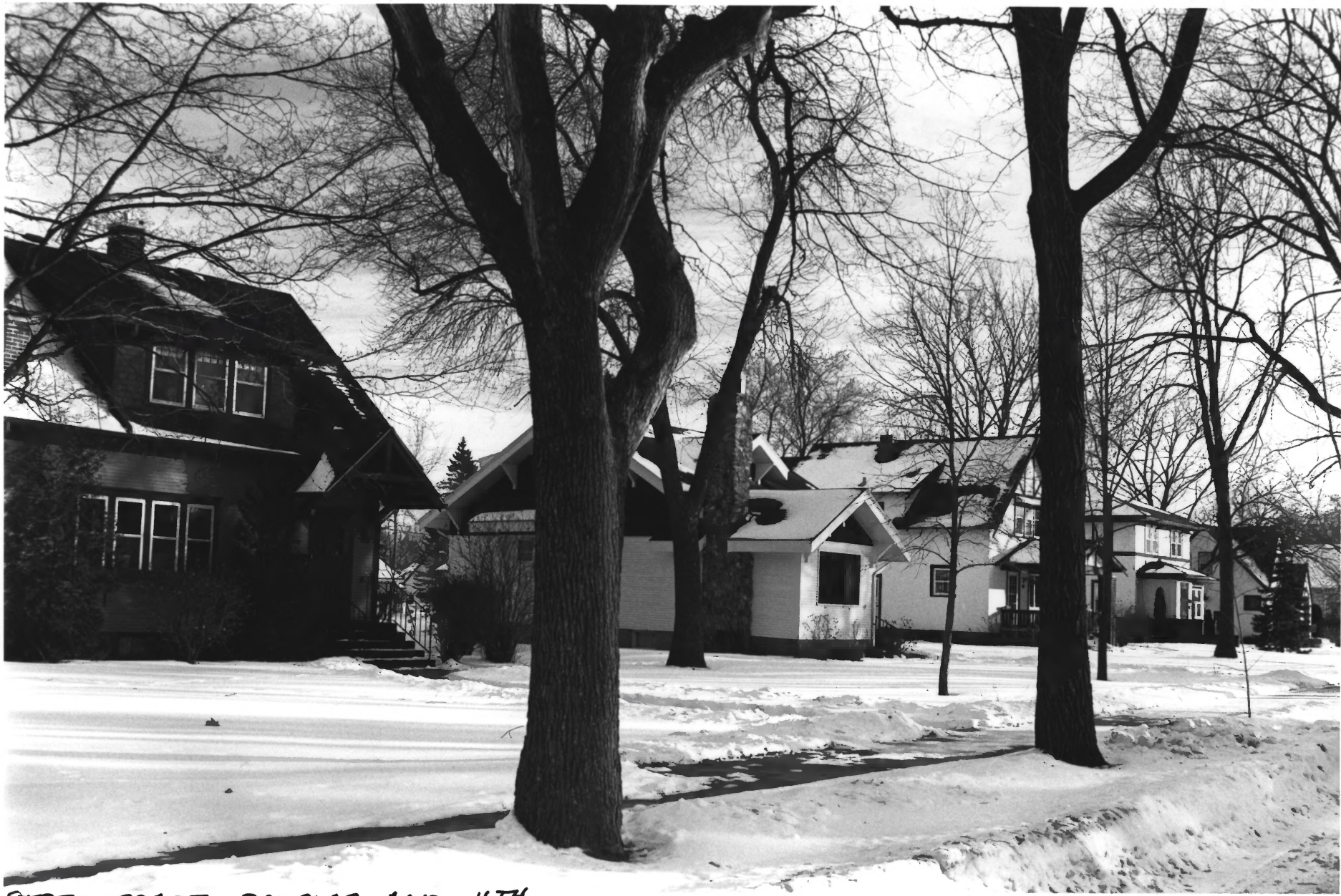
STREETSCAPE : DOUGLAS AND 11 TH ALEXANDRIA RESIDENTIAL HISTORIC DISTRICT ALEXANDRIA, DOUGLAS CO., MINNESOTA 010695 #10
