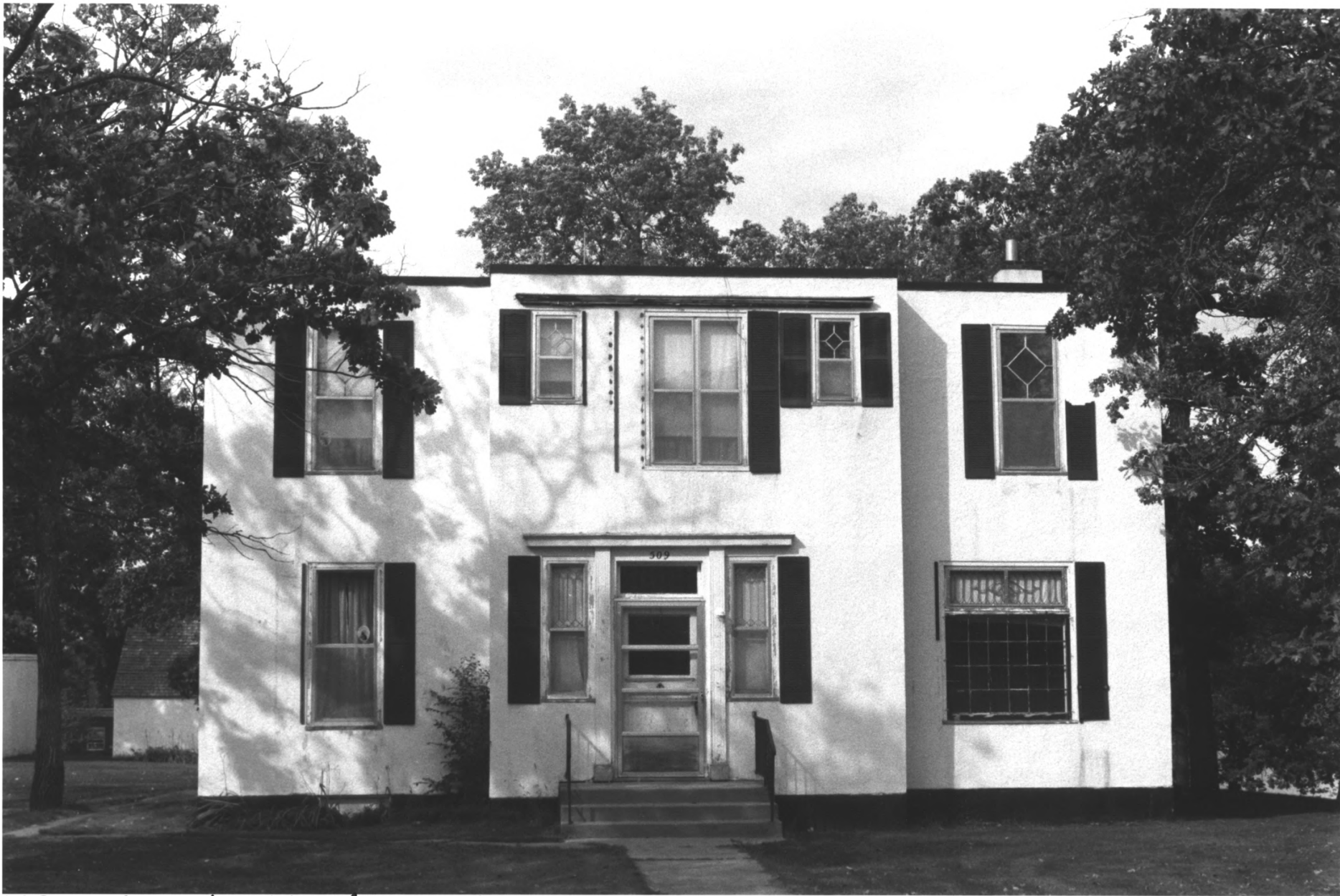
509 LINCOLN AVE. W., BARNES HOUSE ALEXANDRIA RESIDENTIAL HISTORIC DISTRICT ALEXANDRIA, DOUGLAS CO., MINNESOTA 010 632 #11 NON-CONTRIBUTING
