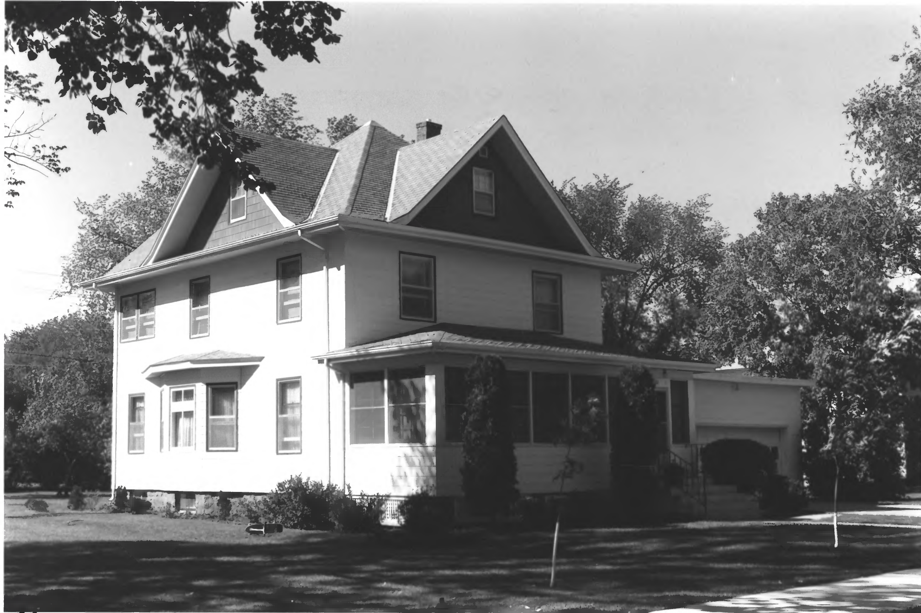
1122 DOUGLAS ST. ALEXANDRIA RESIDENTIAL HISTORIC DISTRICT ALEXANDRIA, DOUGLAS CO., MINNESOTA 010608 #16
