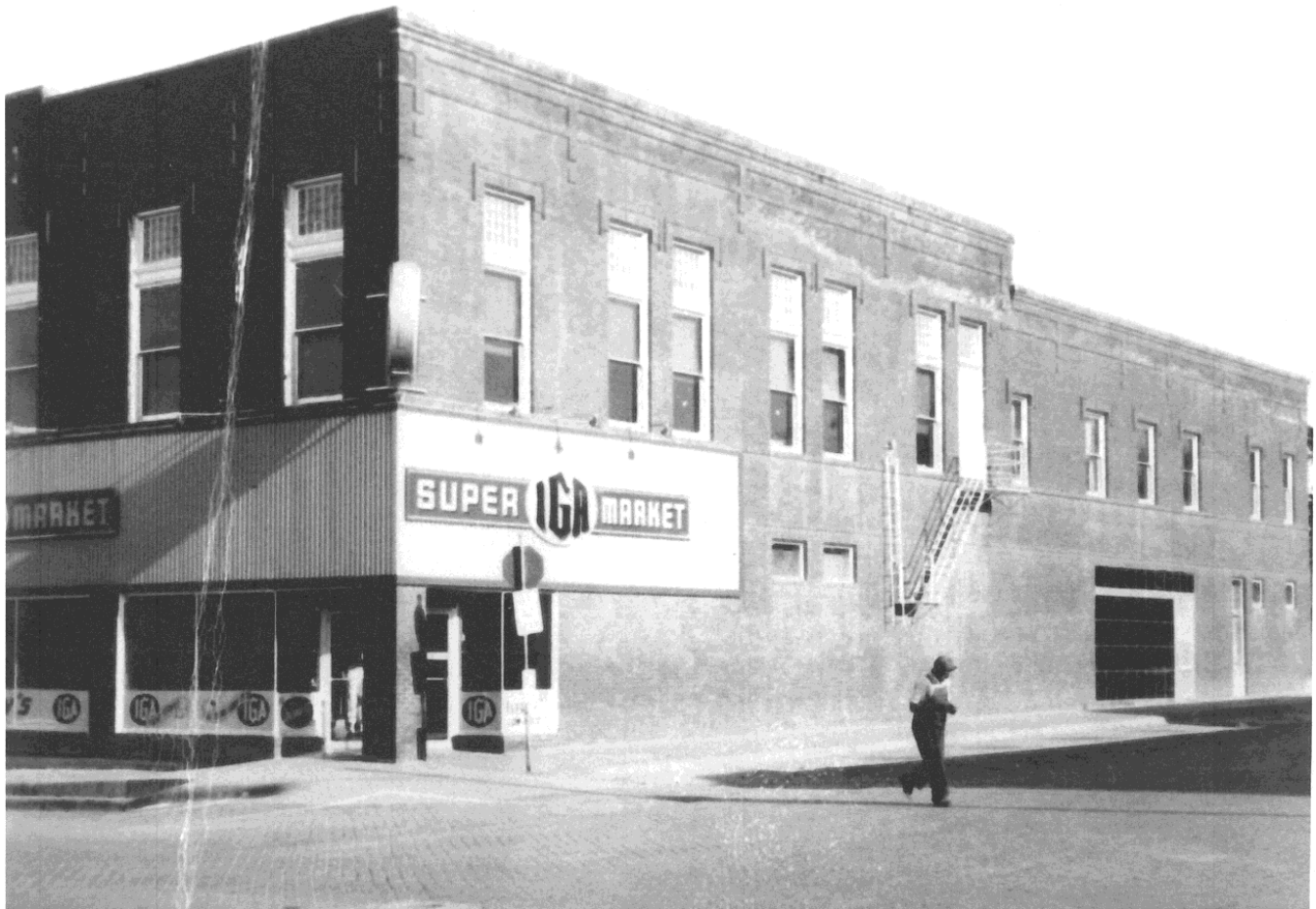
Figure 5: 1950s view of north (left) and west facades, view facing southeast. Owner's collection.
