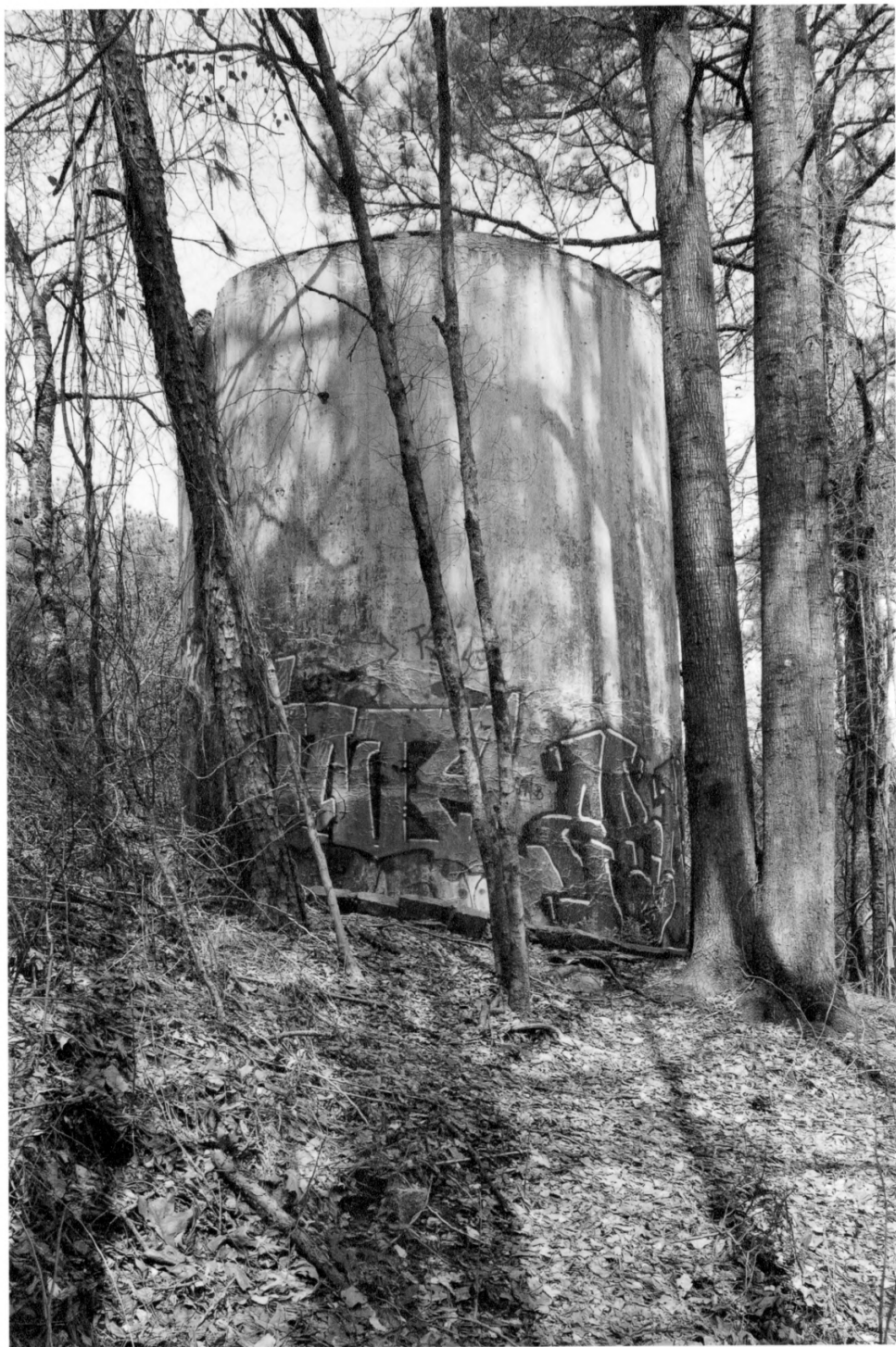
Decatur Waterworks DeKalb County, Georgia Photograph | 9 of 33
