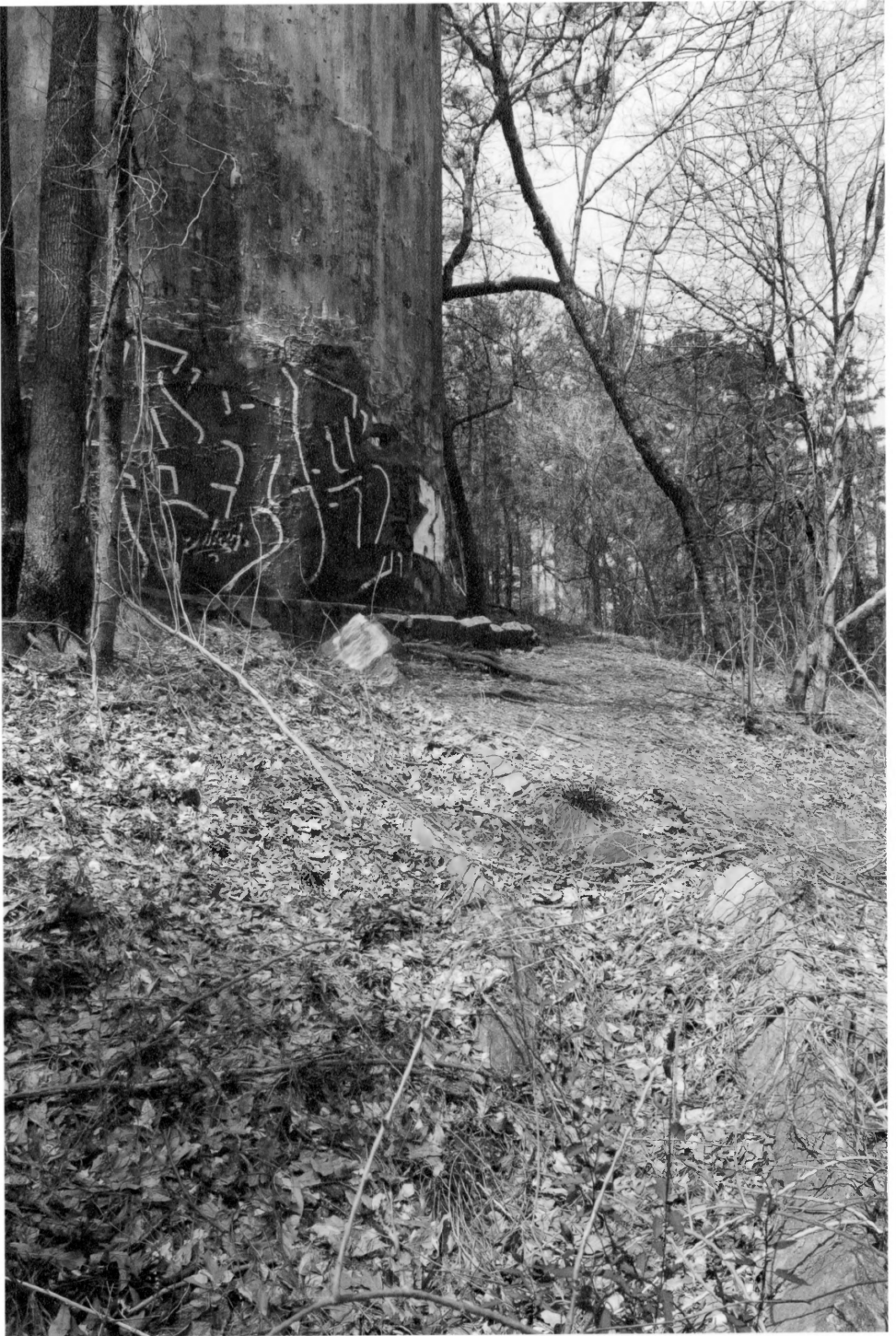
Decatur Waterworks DeKalb County, Georgia Photograph 20 of 33
