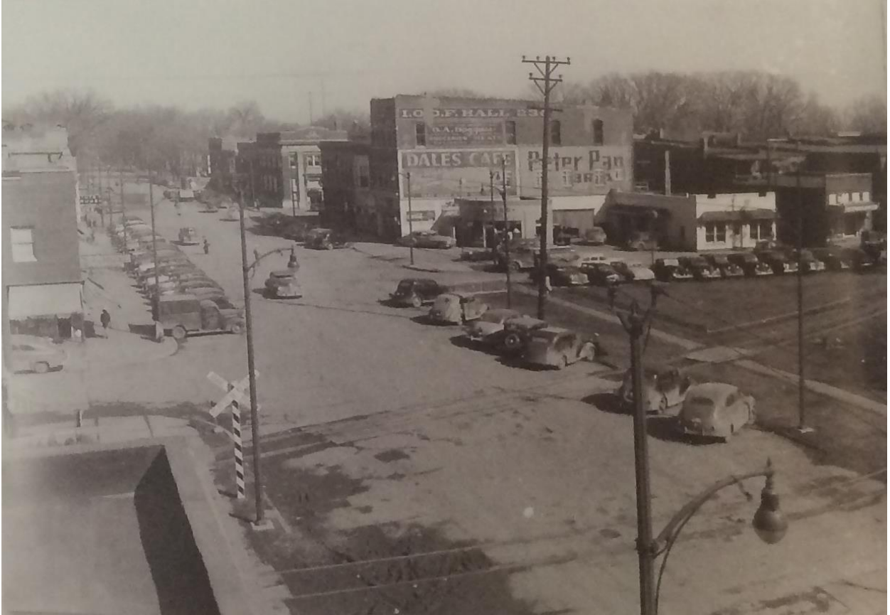
Description of Photograph(s) and number, include description of view indicating direction of camera: South College Avenue looking northeast from the roof of a building on the 200-Block. 12 of 30.
