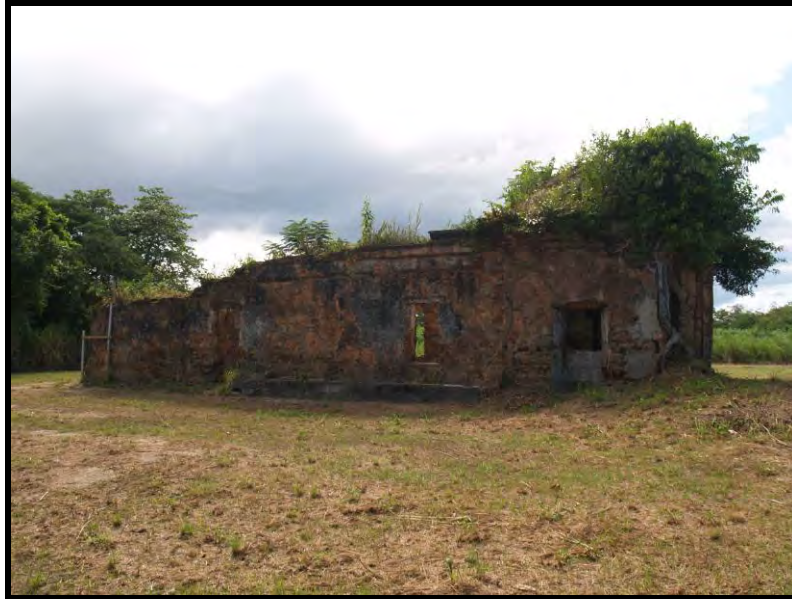
Figure 8. View of east façade. (Photographer: José Marull)
