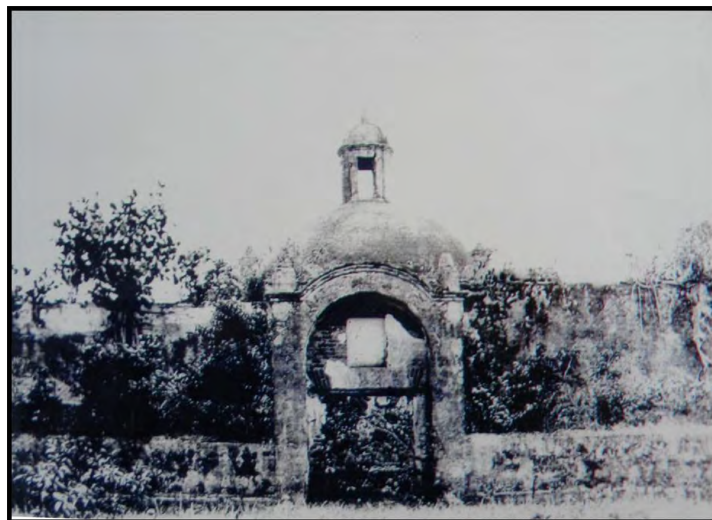
Figure 13. Historic photograph of the cemetery gate and wall and view of the hermitage's cupola and lantern. 41
