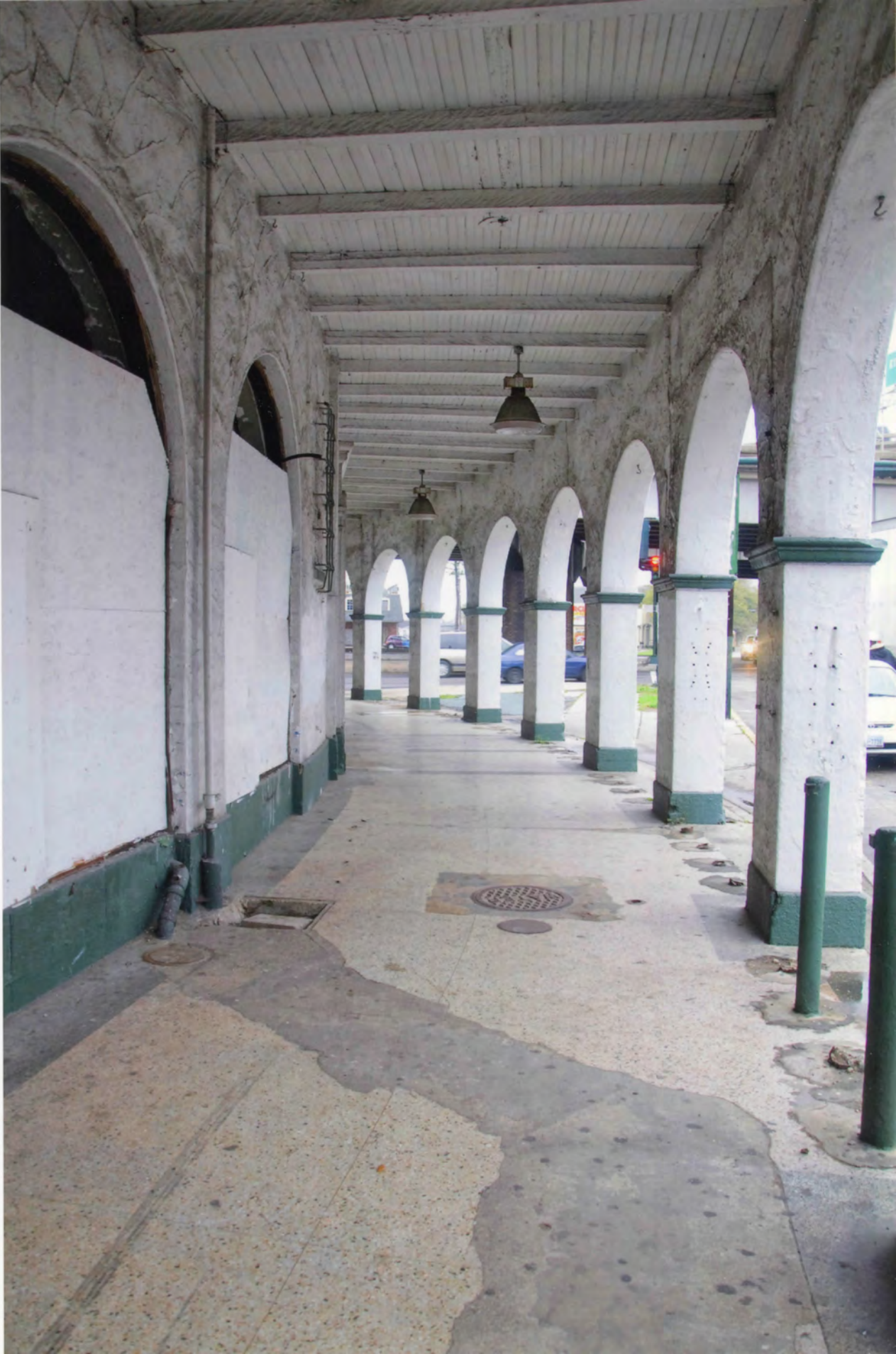
St. Bernard Market New Orleans Orleans Parish Louisiana Photographer John Williams February 2012 St. Bernard Arcade - Camera Facing NW Photo 0002
