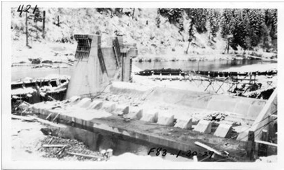
Figure 14: Upstream Face of Roller Gate No. 3 during dam construction, January 30, 1929 (EWEB Archive No. 419)
