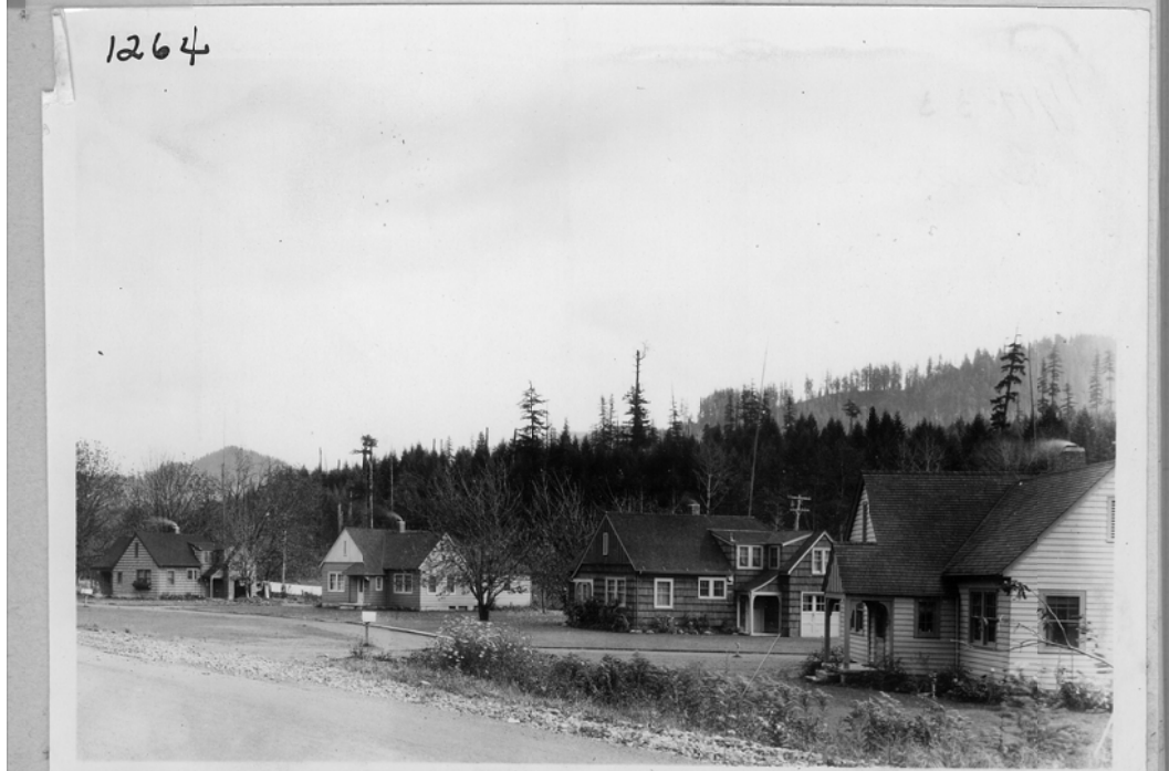
No. 1264 - Taken by H. P. Currin - Nov. 17, 1933 - Leaburg Operators' Houses.
