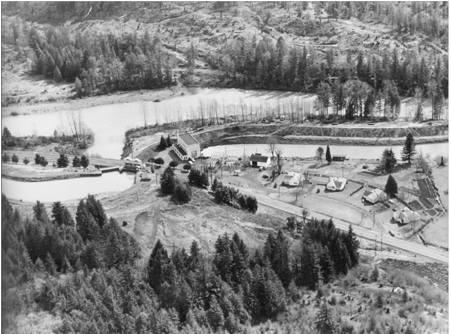
Figure 23: Leaburg Powerhouse and Leaburg Village aerial view, 1937; Canal and Penstock Headgates at left, Tailrace exiting the Powerhouse to the right, south of the housing area (EWEB Archive)
