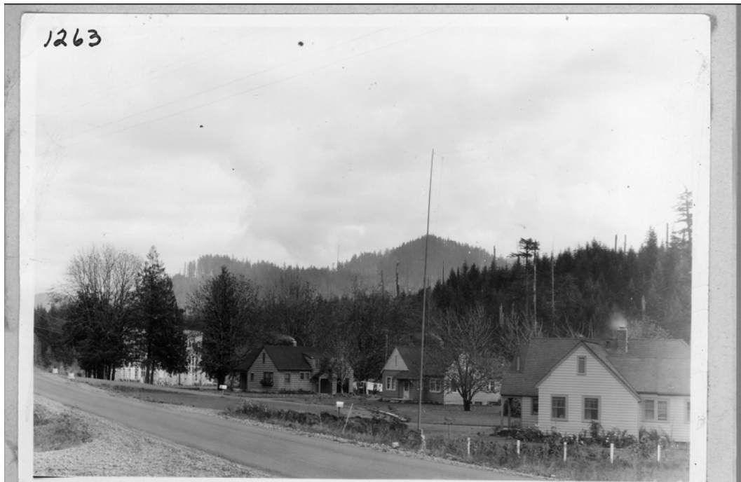
No. 1263 - Taken by H. P. Currin - Nov. 17, 1933 - Leaburg Operators' Houses.
