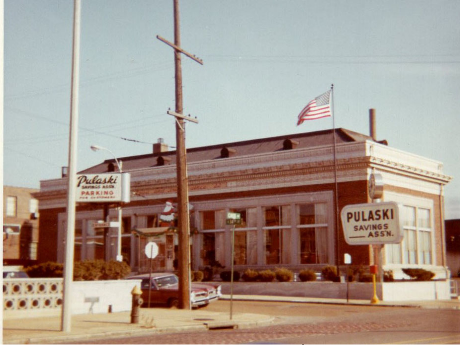
Figure 3. Crunden Branch Library, c. 1970, Cass Avenue and N. 14 th Street, view is northeast from Cass Avenue. The building was used as a bank after it closed as a library in 1954 (Photo Courtesy of Landmarks Association of St. Louis, Inc., 911 Washington Avenue, St. Louis, MO).
