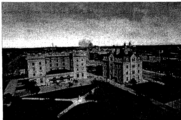
Postcard view of new Post Office (left) and converted City Hall (right), ca. 1910.
