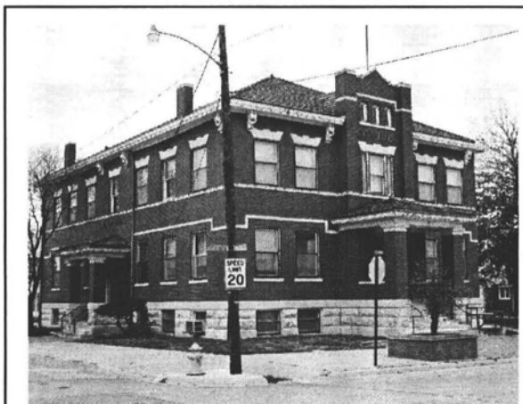
Old Ottawa City Hall 123 West 4 th Street
