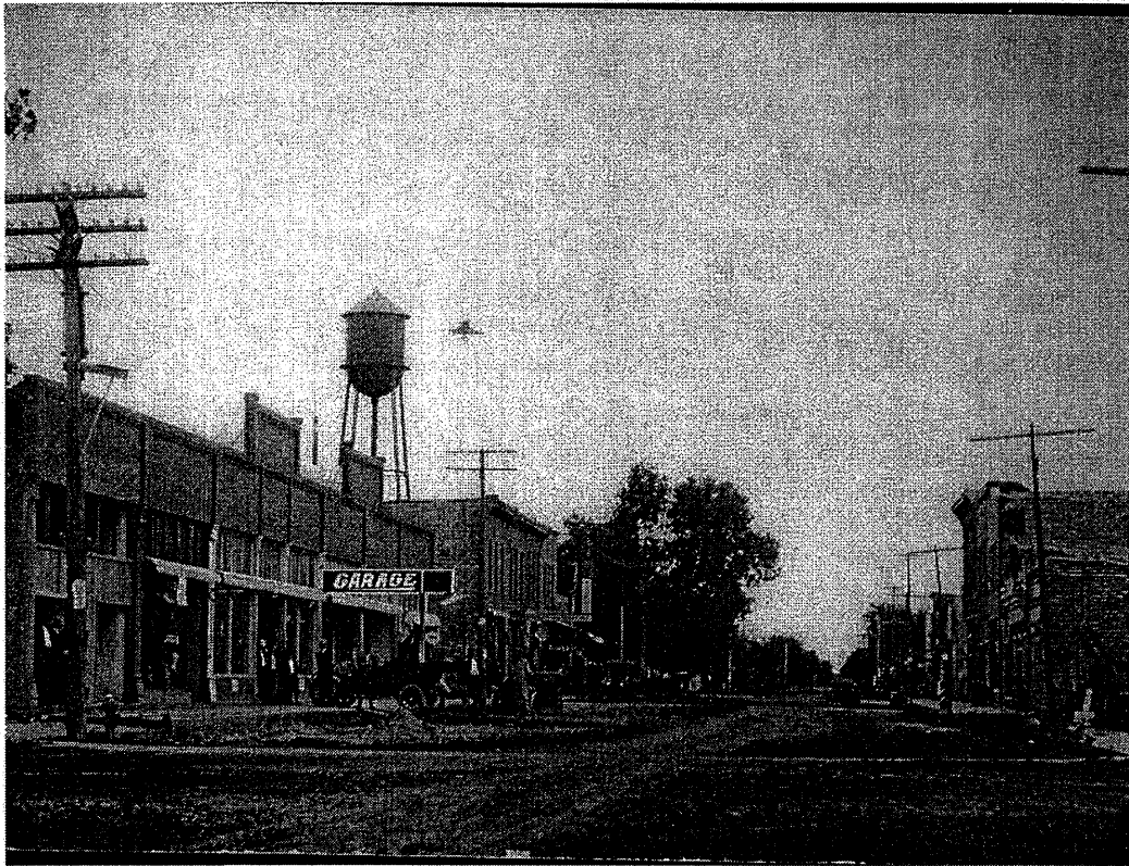
C: Main Street, c.1912, looking east
