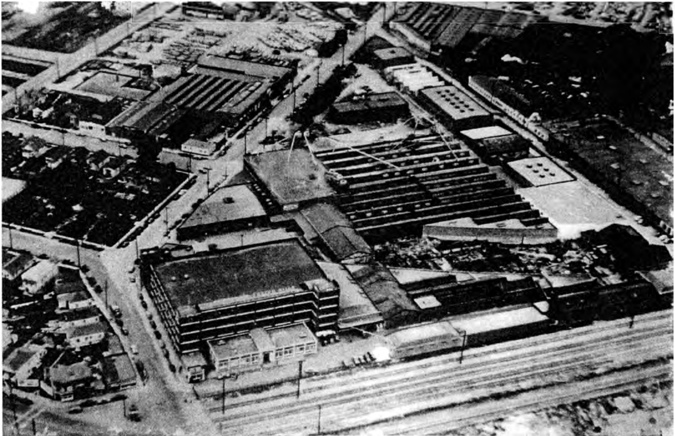
Figure 9. Aerial photograph, Nimitz freeway (I-880) under construction, 1953 or earlier. Image courtesy OCHS.
