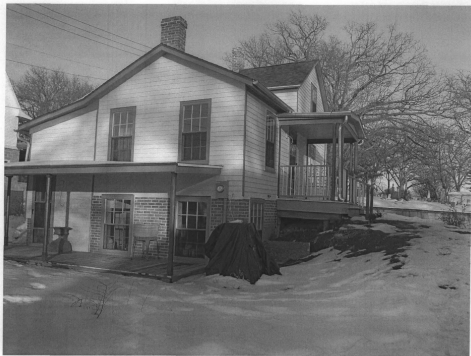
Illustration #16: West (formerly south) façade of Isaac A. Wetherby House at new location, 611 North Governor Street, Iowa City, Iowa, photographed by Mary Bennett, January 22, 2009.
