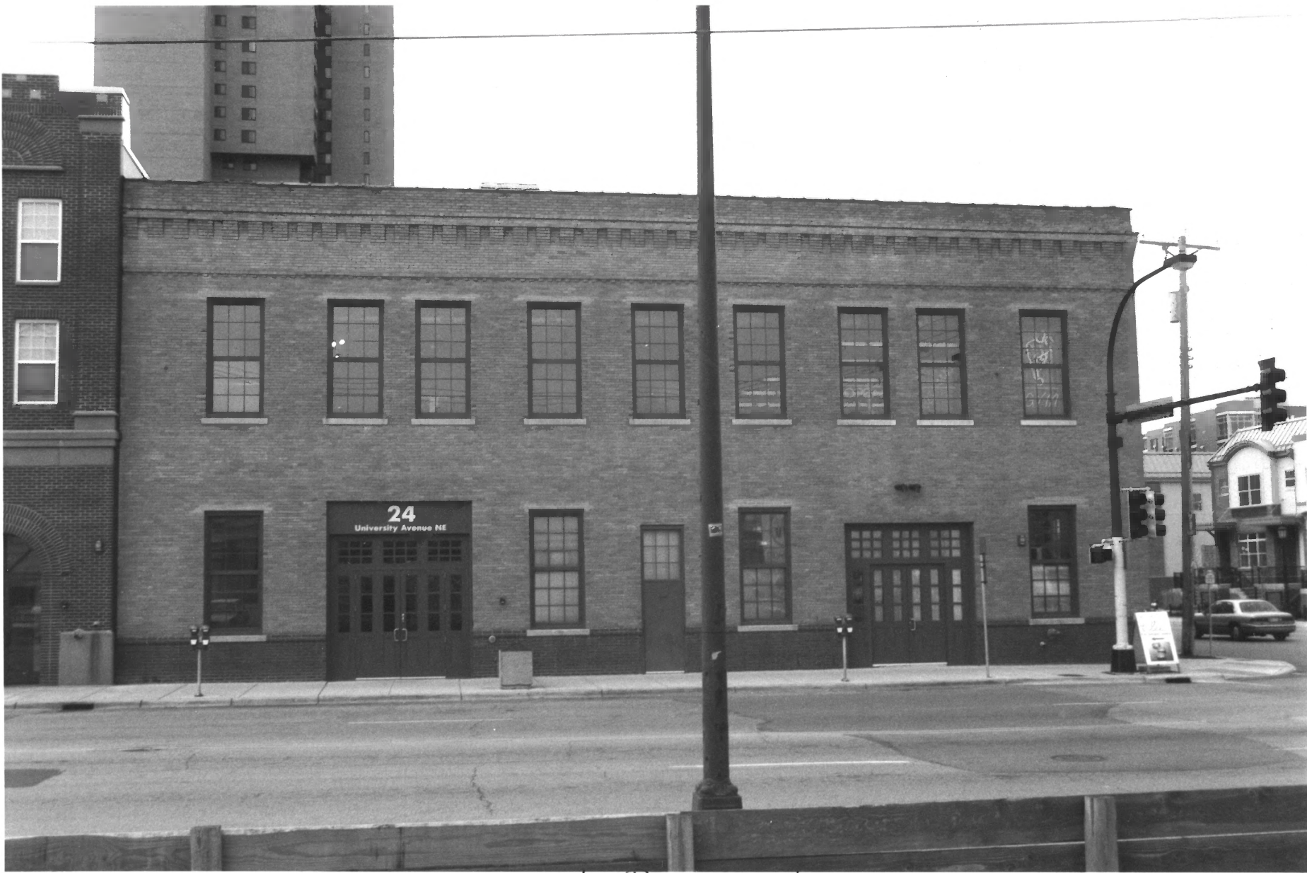
Minneapolis Fire Department Repair Shop Hennepin Co., MN 0148:8-21A
