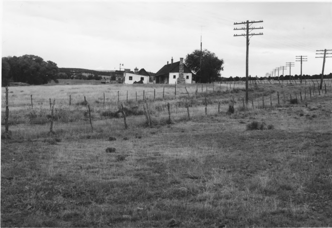
Sapello Stage Station from northeast, at original junction of Mountain and Cimarron Branches. (NPS photo by W. Brown, Oct. 1962; negative in Southwest Regional Office).
