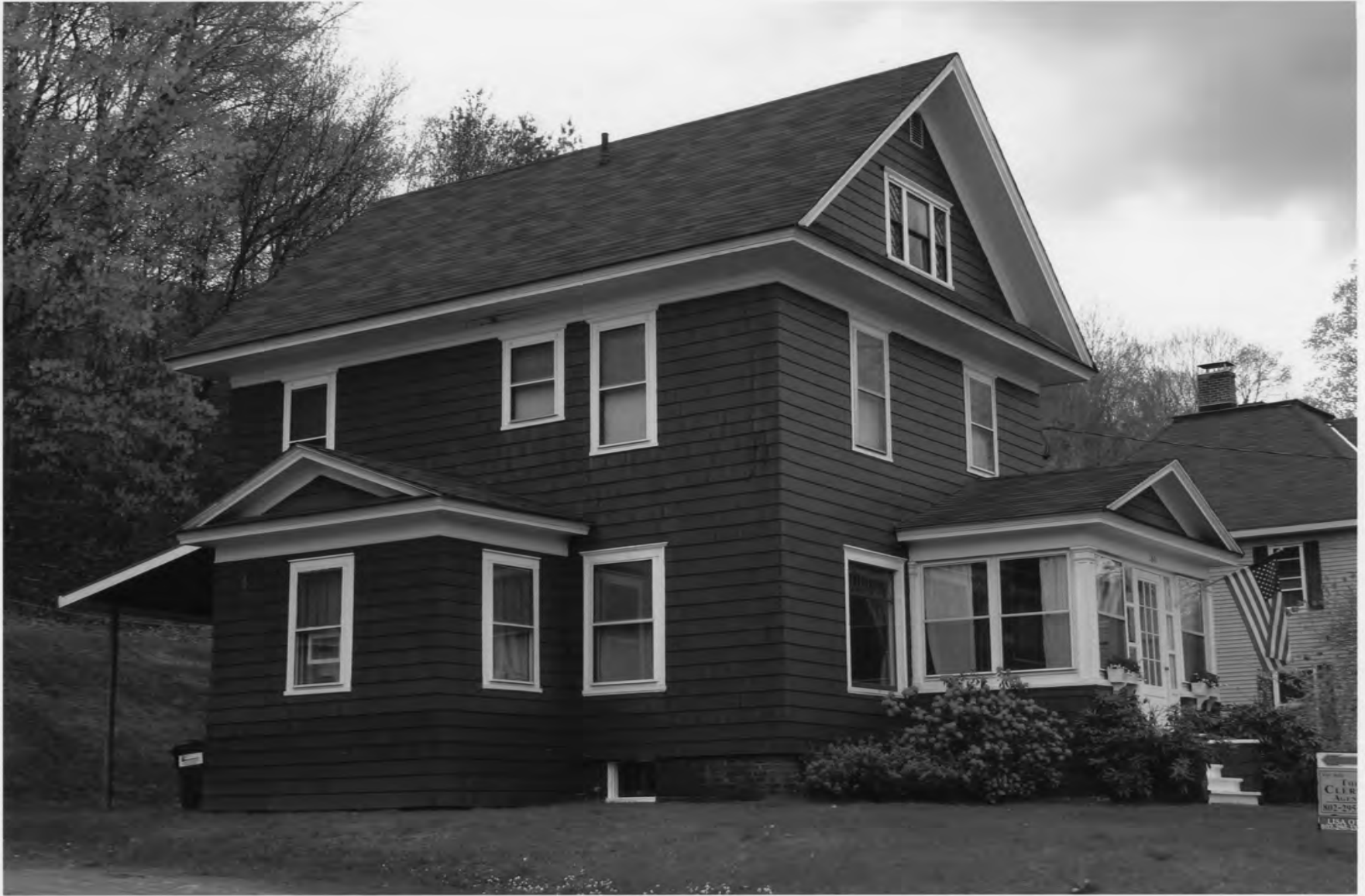
Photograph 34 of 57 Property #25, 260 Fairview Terrace view W. Photographer: Liisa Reimann, May 8, 2011
