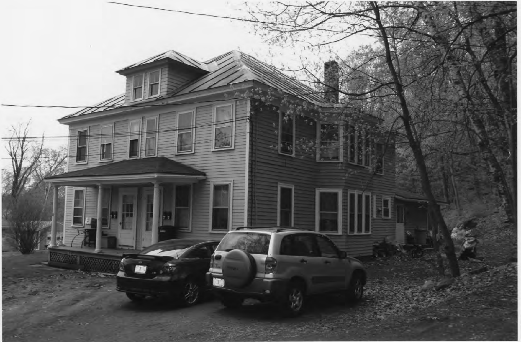
Photograph 55 of 57 Property #45, 38 Hillcrest Terrace, view SW. Photographer: Liisa Reimann, May 8, 2011
