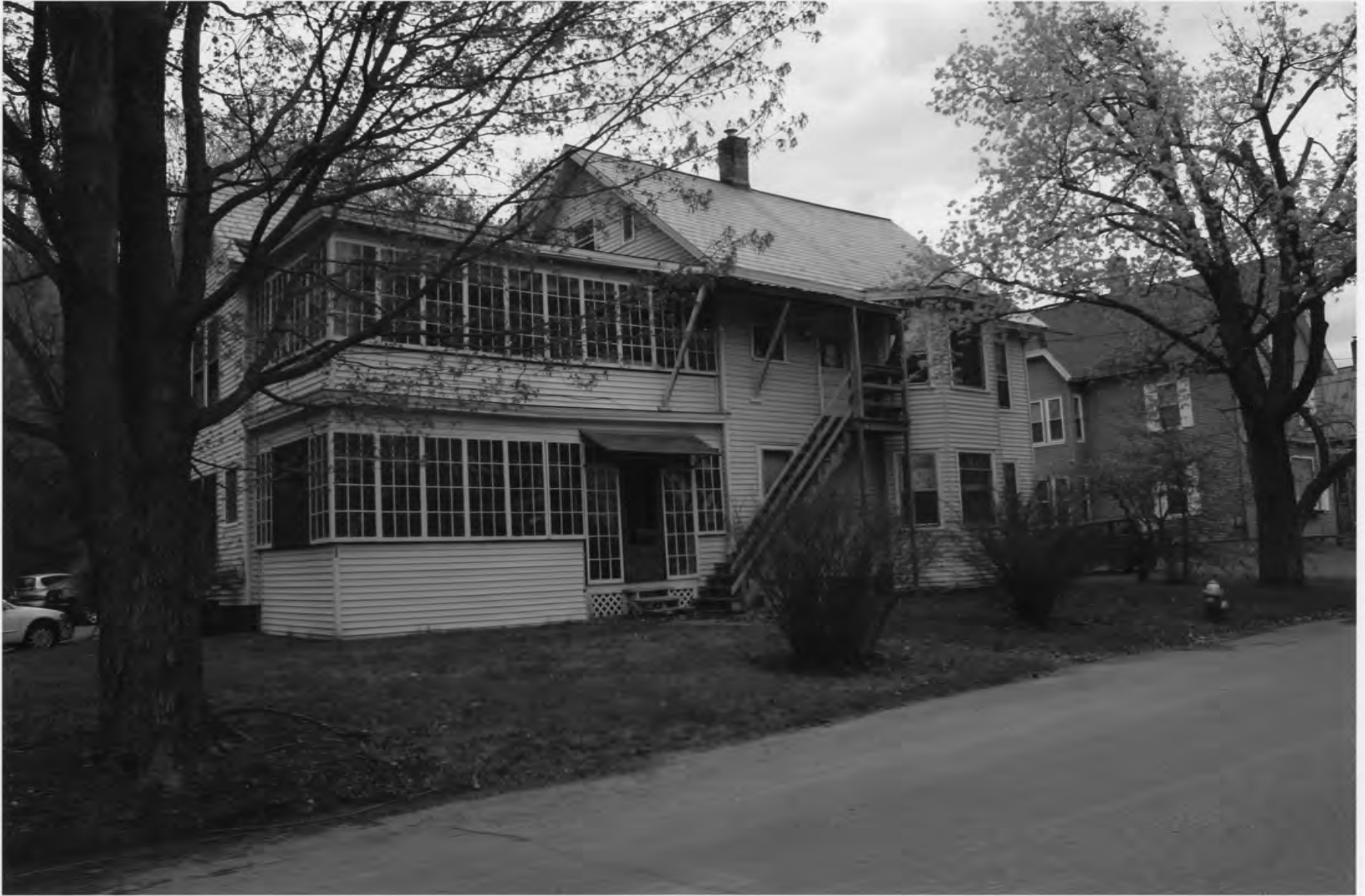
Photograph 12 of 57 Property #4, 22 Maplewood Terrace view NW. Photographer: Liisa Reimann, May 8, 2011
