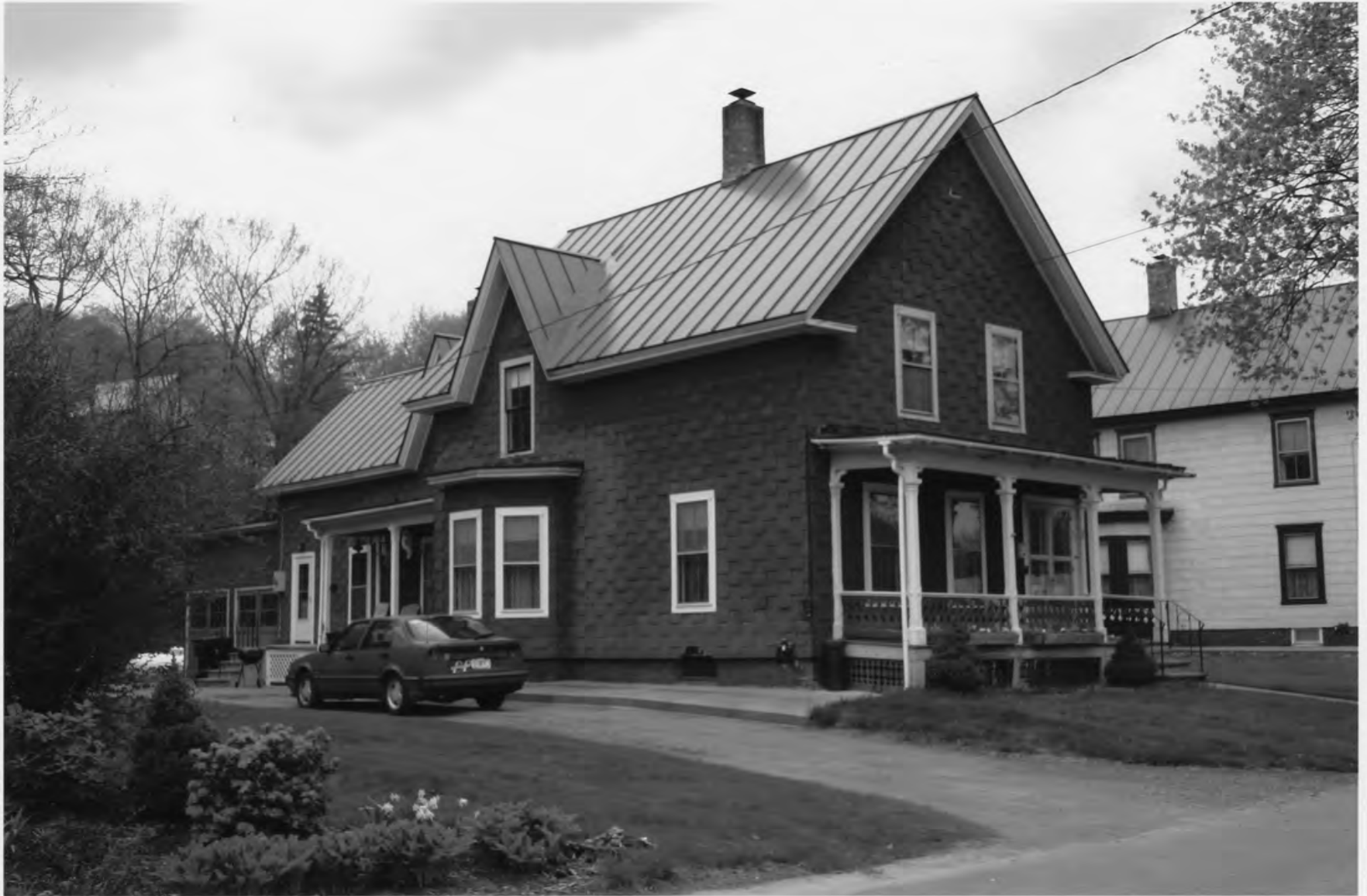
Photograph 10 of 57 Property #2, 56 Maplewood Terrace view NW. Photographer: Liisa Reimann, May 8, 2011
