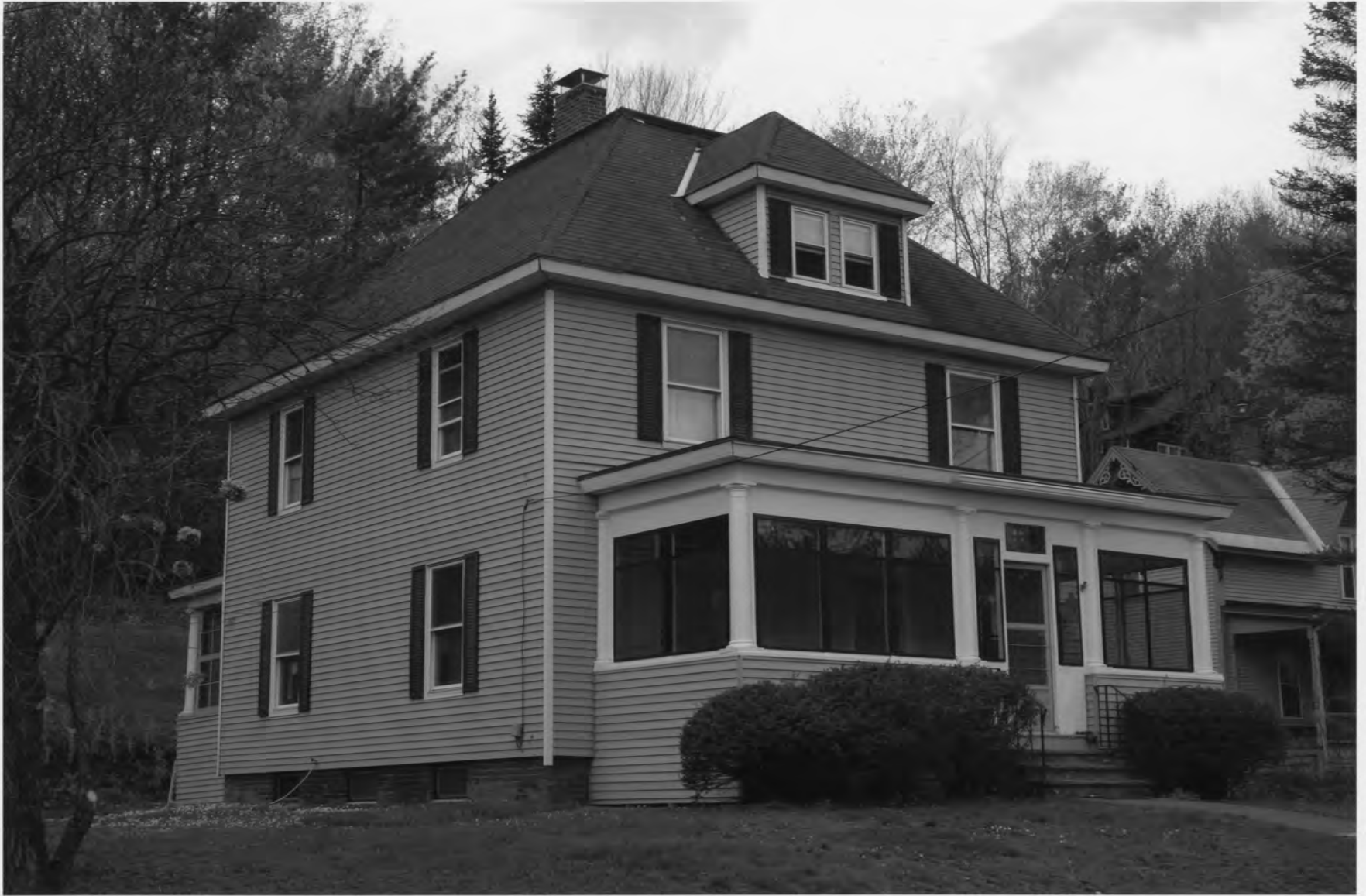
Photograph 35 of 57 Property #26, 278 Fairview Terrace view W. Photographer: Liisa Reimann, May 8, 2011
