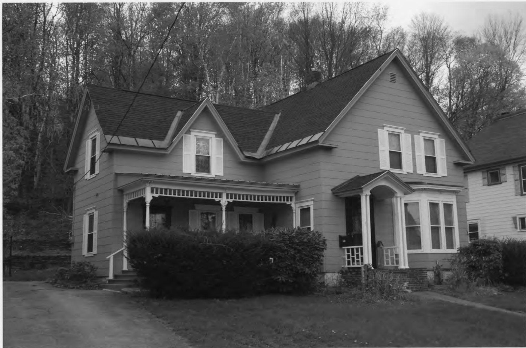
Photograph 32 of 57 Property #23, 234 Fairview Terrace view W. Photographer: Liisa Reimann, May 8, 2011
