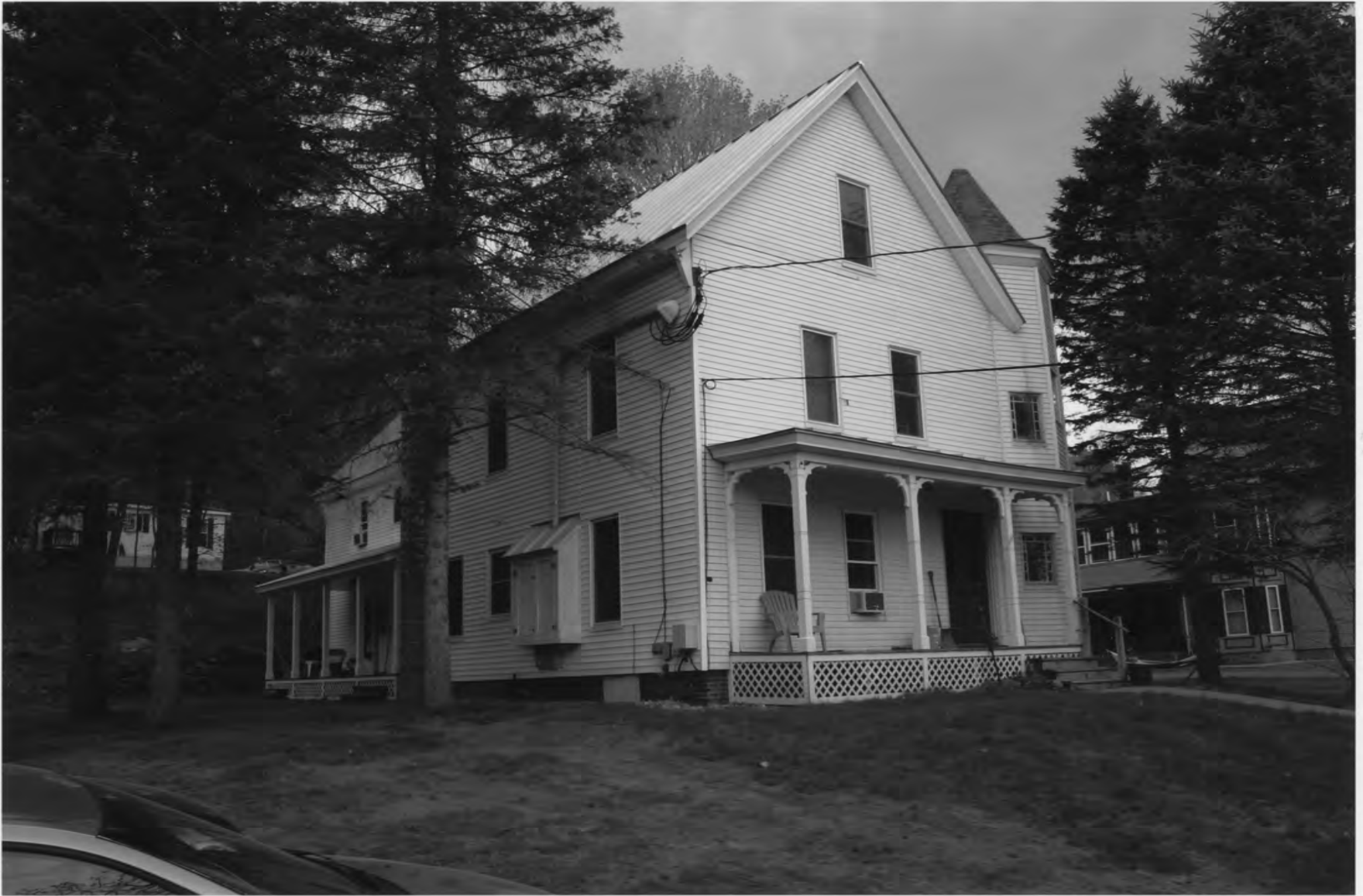
Photograph 22 of 57 Property #13, 122 Fairview Terrace view W. Photographer: Liisa Reimann, May 8, 2011
