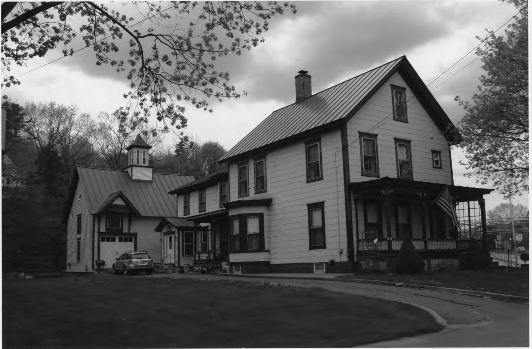
Photograph 9 of 57 Property #1, 60 Maplewood Terrace view NW. Photographer: Liisa Reimann, May 8, 2011
