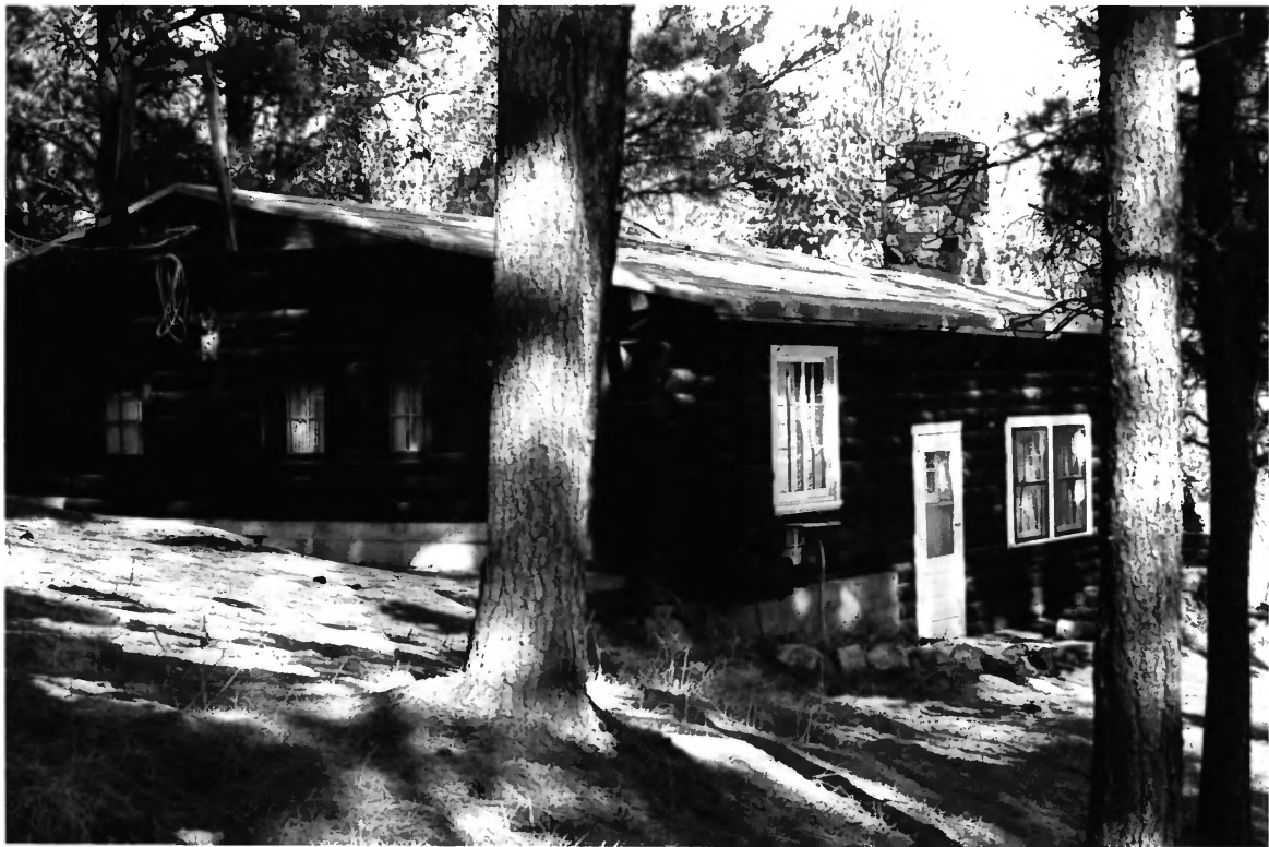
CCC Camp Custer Officers' Cabin , Custer County, S.D. , No. 4
