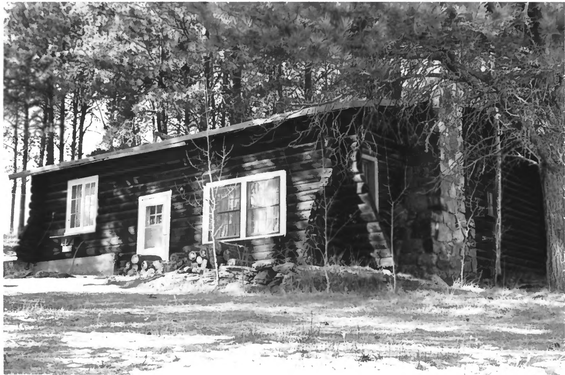
CCC Camp Custer Officers' Cabin, Custer County, S.D., No. 1
