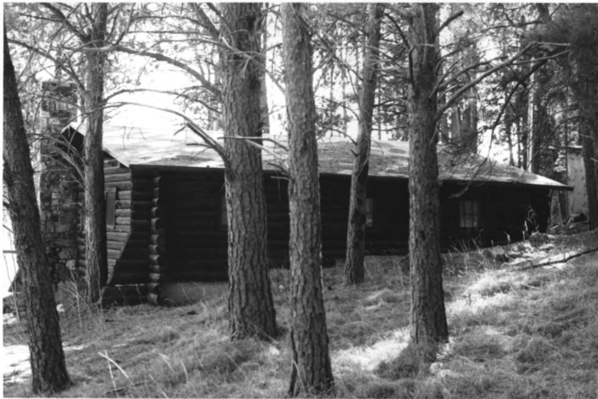
CCC Camp Custer Officers' Cabin, Custer County, S.D., No. 2
