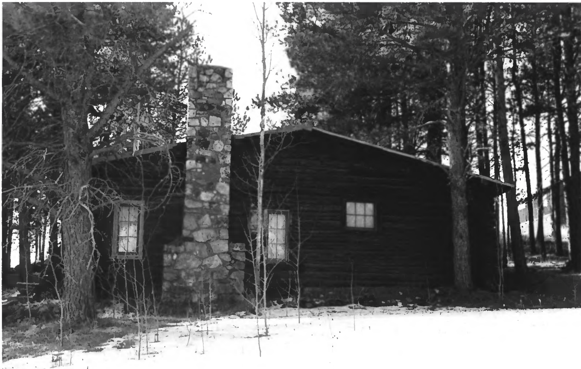
CCC Camp Custer Officers' Cabin, Custer County, S.D., No. 2
