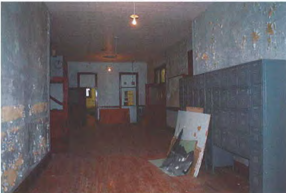
Photograph 16. 1911 Original School - Second Floor, central corridor, looking north
