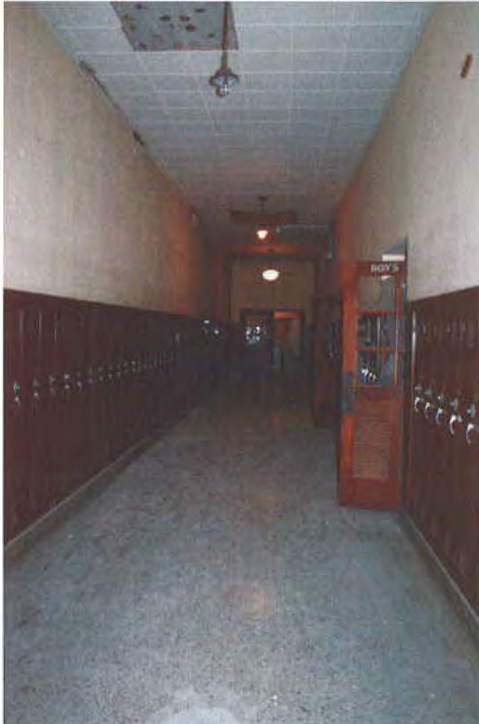
Photograph 22. 1939 Addition - Third Floor, central corridor
