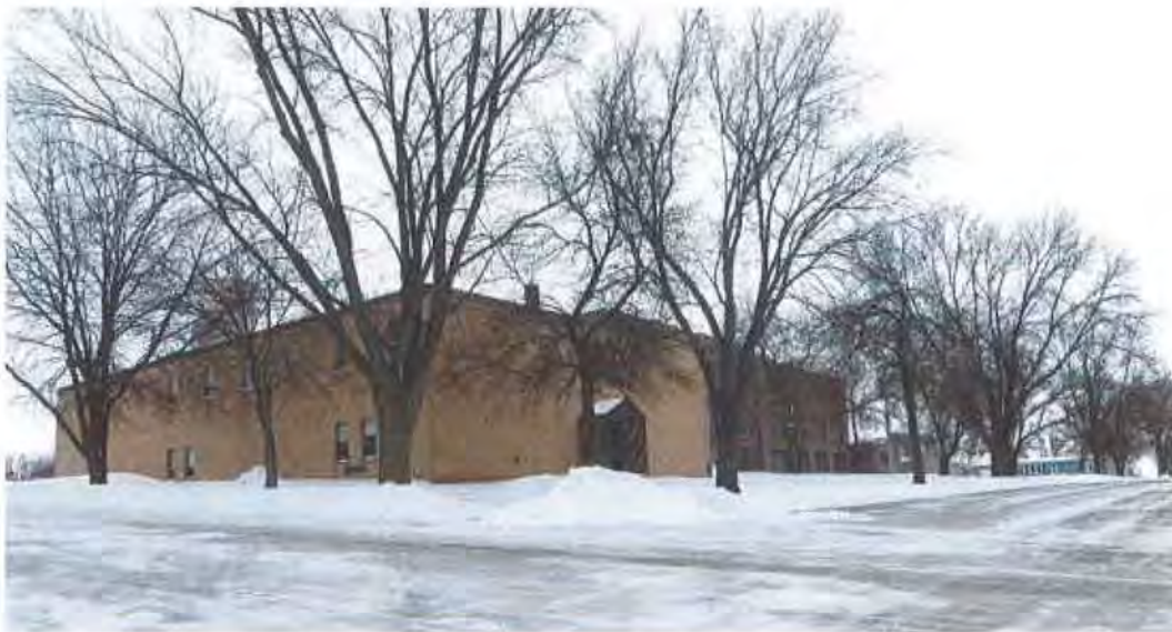
Photograph 02. Jasper School – Site View - 2018
