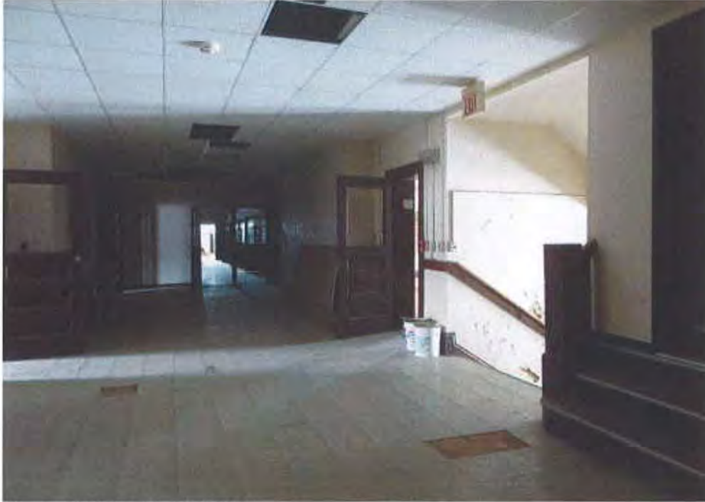
Photograph 15. 1911 Original School - First Floor, central corridor looking south
