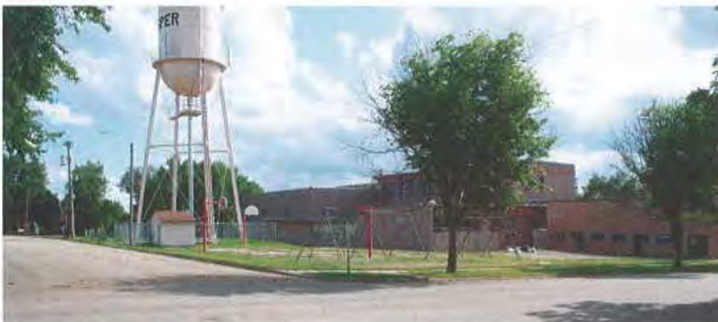
Photograph 03. Jasper School – Site View - 2018
