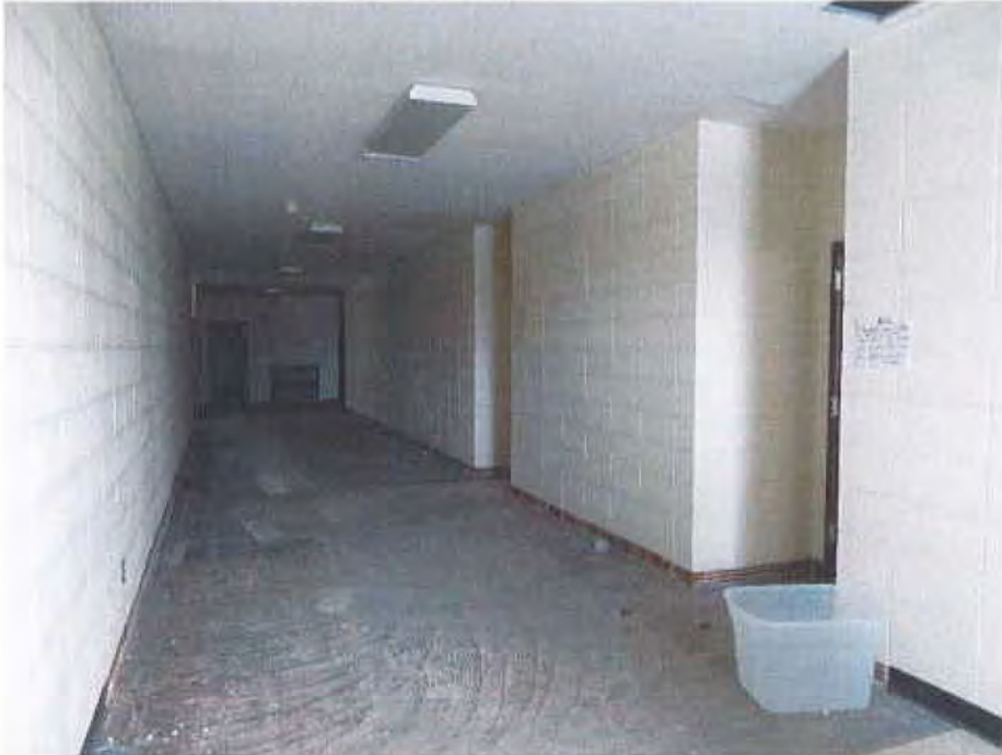
Photograph 29. 1965 Addition - Typical, Double-Loaded Corridor
