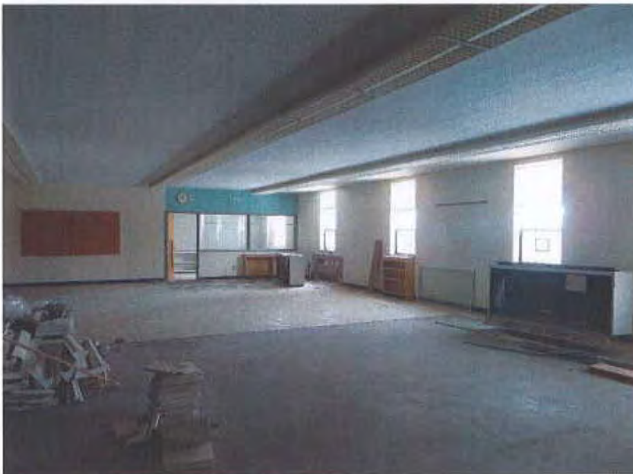
Photograph 30. 1965 Addition - Typical Classroom
