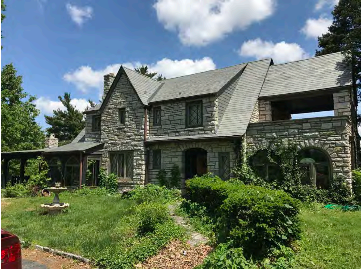
Fig. 41 of 43: Photograph of the main elevation of the Gene Bussen House located at 5501 Remington Villas Ct., Photograph taken by Daniel Gonzales, May 2017
