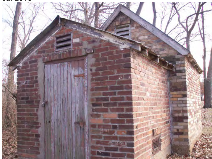
Fig. 31 of 43: Western elevation of smokehouse, camera facing east, Photograph Taken by Nikole Meyer ca. 2016
