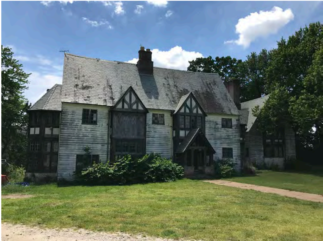
Fig. 42 of 43: Photograph of the main elevation of the Hillcrest Country Club located at 8100 Fine Road. Photograph taken by Daniel Gonzales, May 2017
