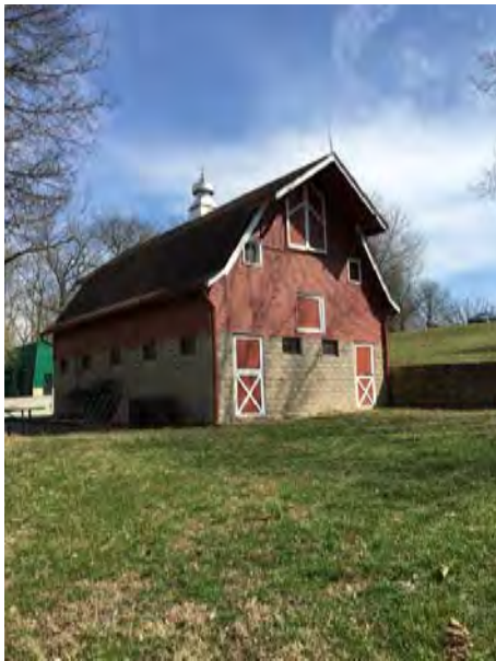
Fig. 33 of 43: Southern elevation of barn, camera facing north, Photograph Taken by Nikole Meyer ca. 2016
