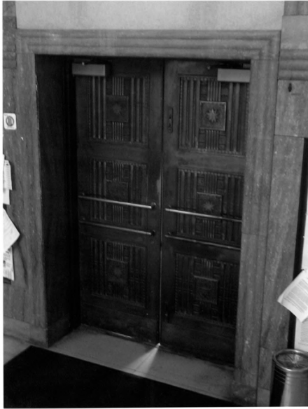
Fountain County Courthouse, Fountain County, IN #20
