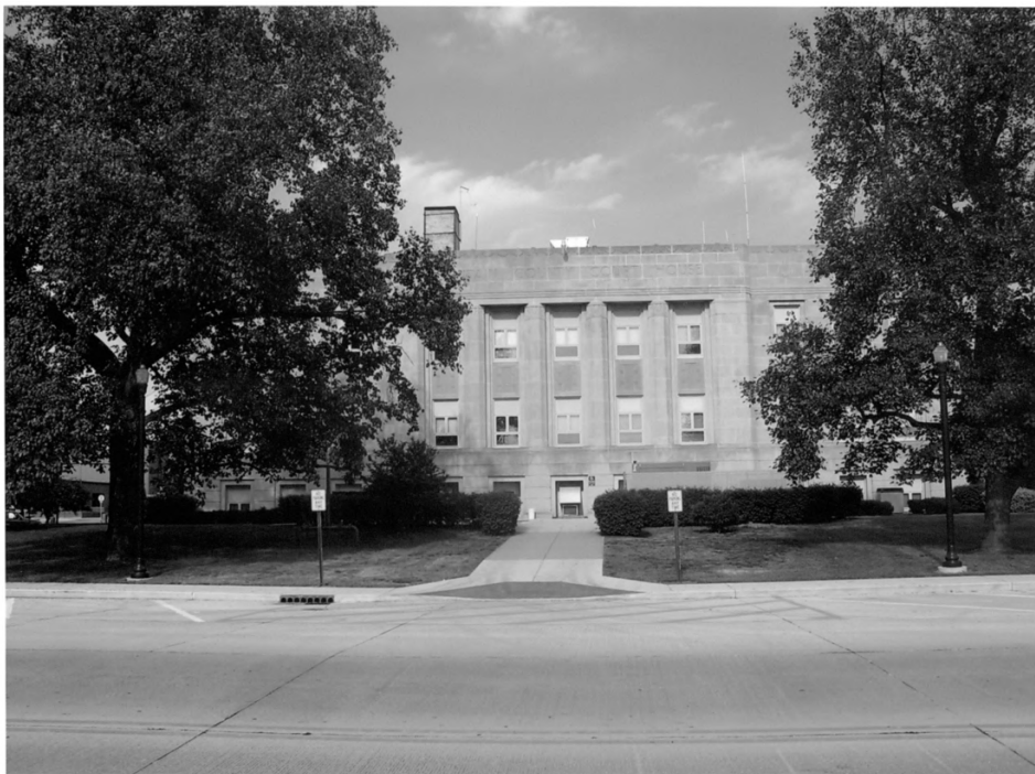
Fountain County Courthouse, Fountain County, IN #6
