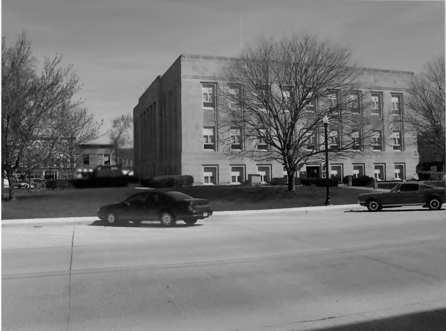
Fountain County Courthouse, Fountain County, IN #5
