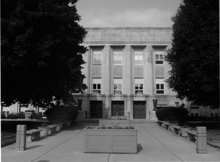
Fountain County Courthouse, Fountain County, IN #1
