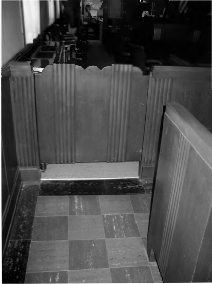
Fountain County Courthouse, Fountain County, IN #19
