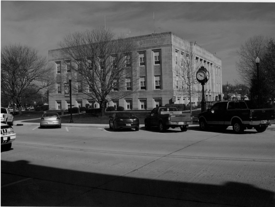
Fountain County Courthouse, Fountain County, IN #4
