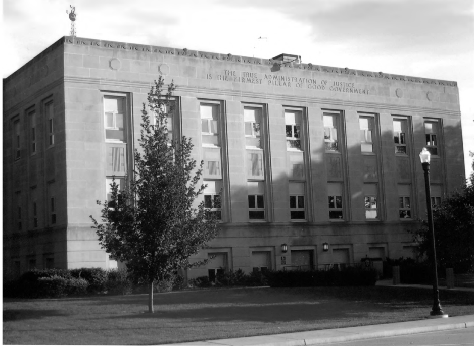
Fountain County Courthouse, Fountain County, IN #7
