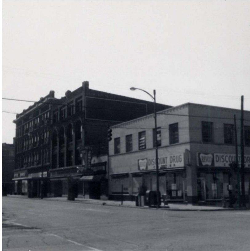
Figure 13. A 1972 photograph showing 1100, 1108, 1118 and 1124 Central Avenue in the Central Avenue Historic District in Middletown, Ohio, looking southwest
