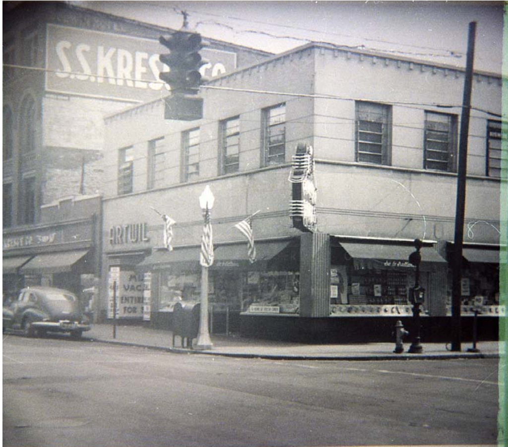
Figure 12. Ca. 1950 photograph of 1100 and 1108 Central Avenue in the Central Avenue Historic District in Middletown, Ohio, looking southeast
