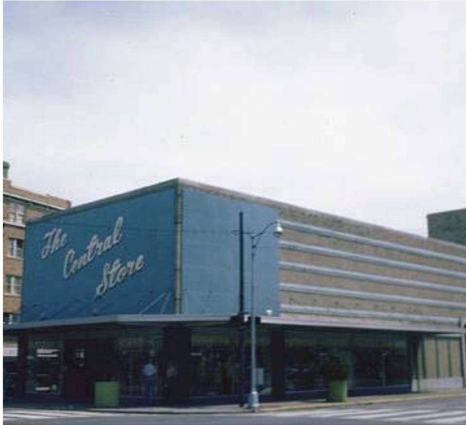
Figure 20. Ca. 1970 photograph of 1150 Central Avenue in the Central Avenue Historic District in Middletown, Ohio, looking southeast
