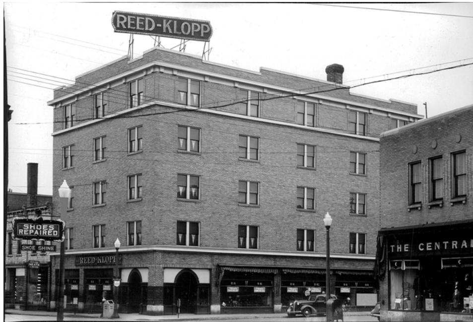
Figure 21. Ca. 1945 photograph of 1200 Central Avenue in the Central Avenue Historic District in Middletown, Ohio, looking southeast
