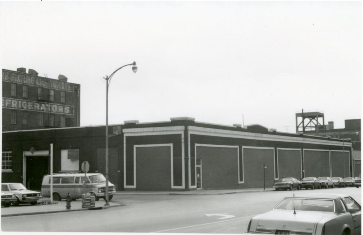
Figure 12. A 1982 photo shows 1701 McGee Street with storefront infill after the Kansas City Star newspaper purchased the building in 1968. Source: Midtown Survey Final Report Kansas City, Jackson County, Missouri, 1981-85. Kansas City Landmarks Commission, Kansas City, Missouri, 2008, survey form JA-A3-008-1219.
