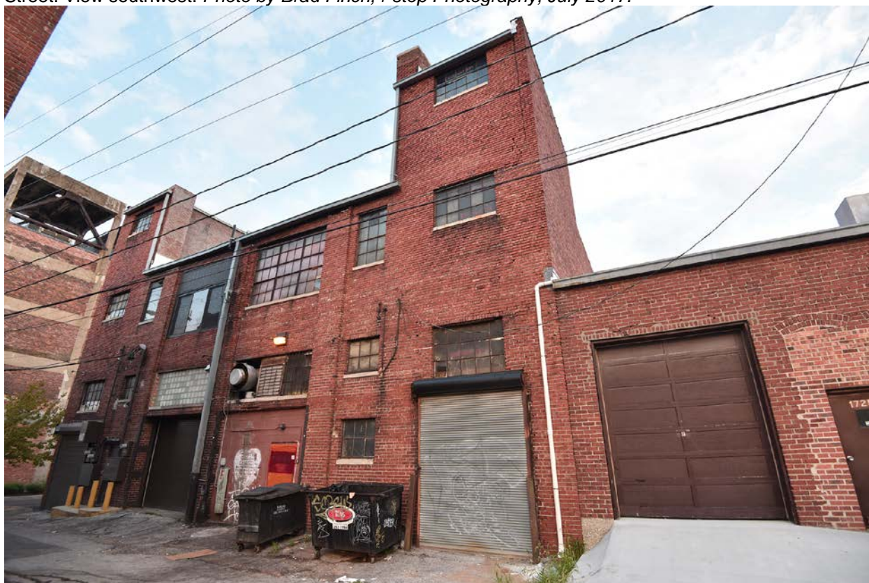
Figure 9. Elevator shaft and vehicular entrances on the rear elevation of 1727 and 1729 McGee Street. View southwest. Photo by Brad Finch, f-stop Photography, July 2017.
