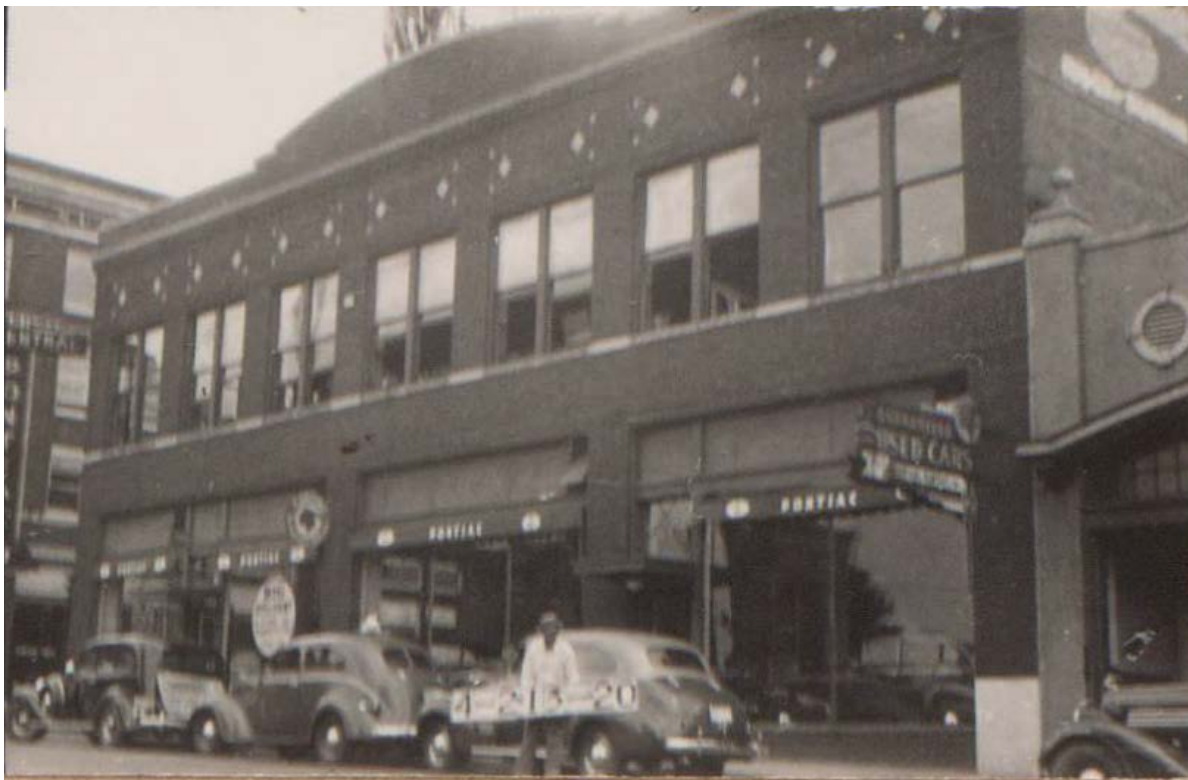
Figure 10. 1801 McGee Street had large storefront glazing on the ground floor showroom space. Source: Kansas City 1940 Tax Assessment Photograph, Missouri Valley Special Collections, Kansas City Public Library, Kansas City, Missouri.
