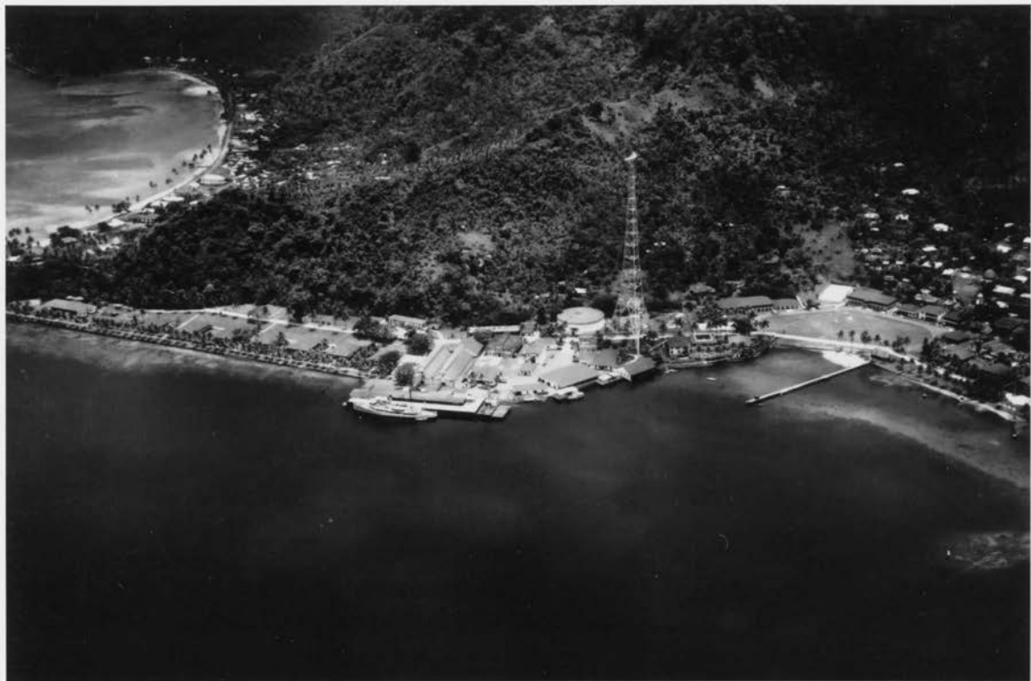
#1. VIEW OF U.S. NAVAL STATION, 1988, TUTUILA ISLAND AMERICAN SAMOA
