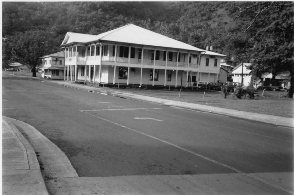
#8. ADMINISTRATION BUILDING, NAVY NO. 21, 1988, U.S. NAVAL STATION TUTUILA, AMERICAN SAMOA
